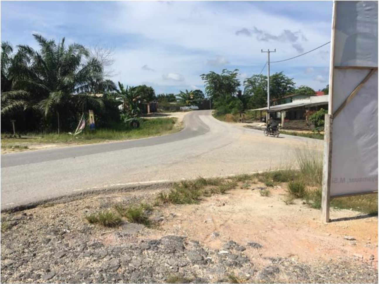
Figure 16.4 : Road Crossing at Tualang Timur Village
