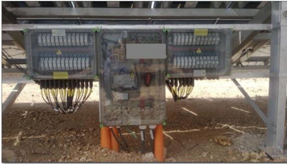
Figure 13. String monitoring unit
