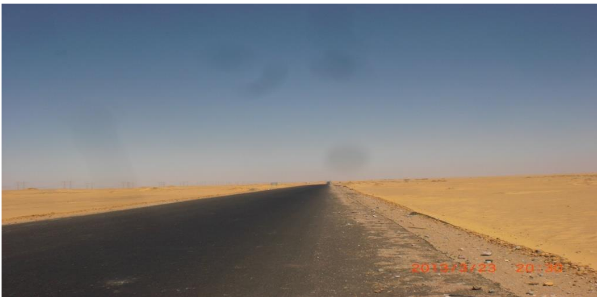
Figure 64. Aswan – Luxor Highway
