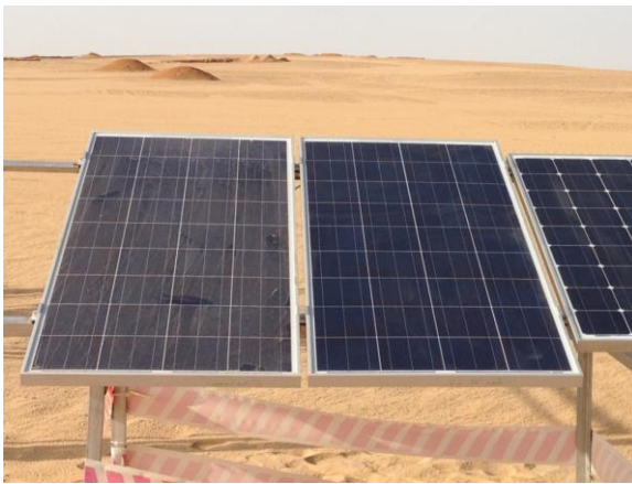
Figure 67: Trial panels at Benban
