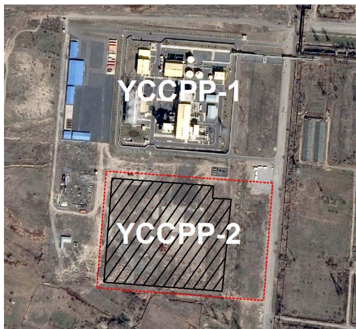
Figure 1-1: Site location (red) of the planned YCCPP-2 (black), next to the existing YCCPP-1
