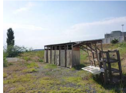
Figure 6-5: Old changing rooms and wash basins
