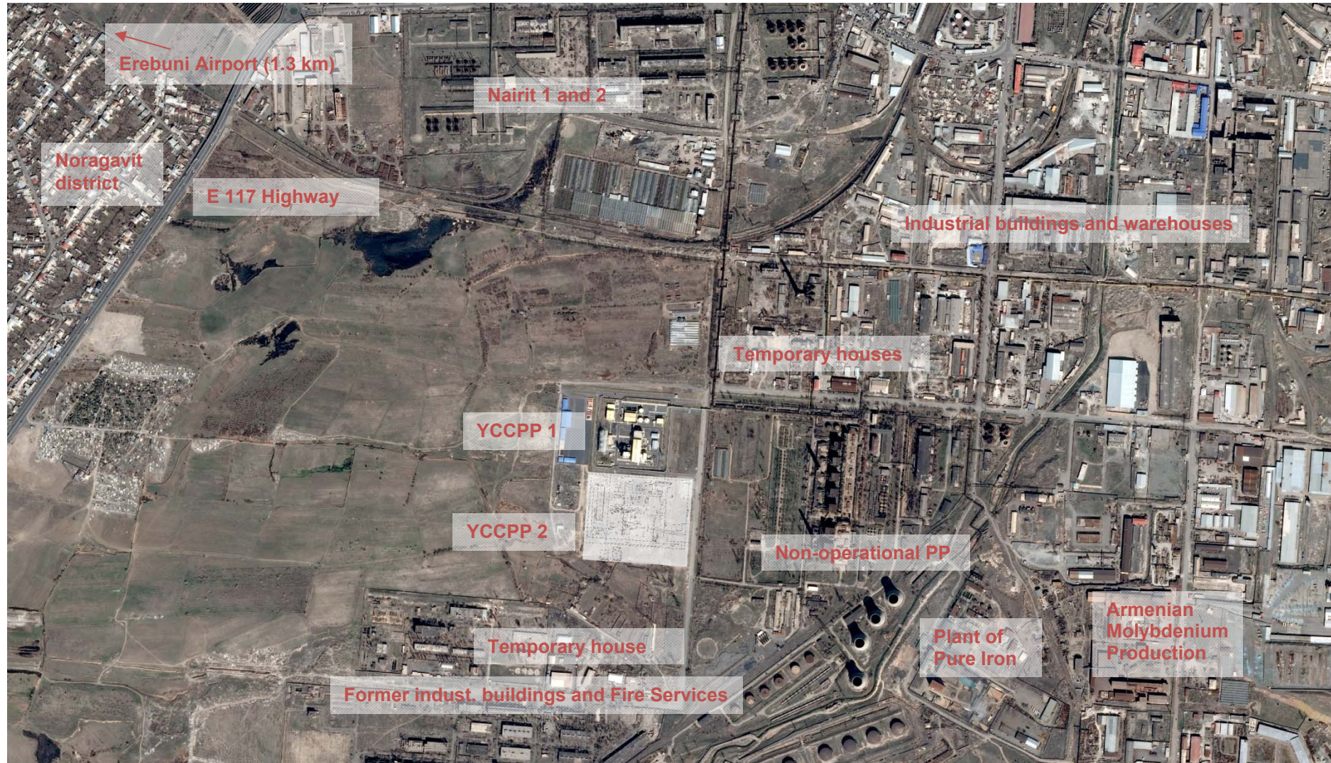
Figure 2-2: Overview of the immediate surroundings of the Yerevan Power Plants 1 and 2
