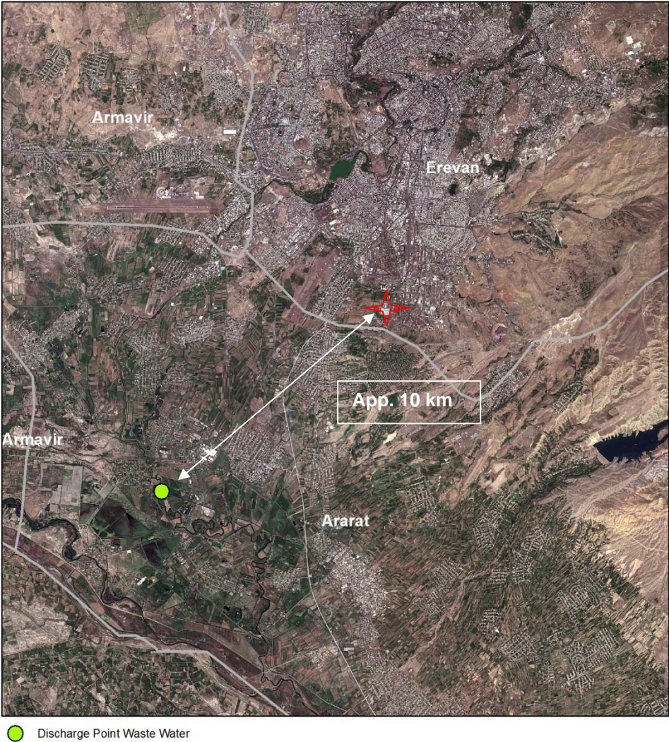
Figure 5-3: Discharge point for the waste water from YCCPP-2
