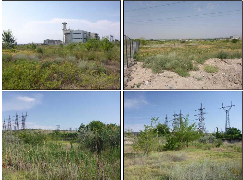
Figure 5-1: Typical vegetation at the construction site with some reed and bushes (Source: Fichtner, July 2017)
