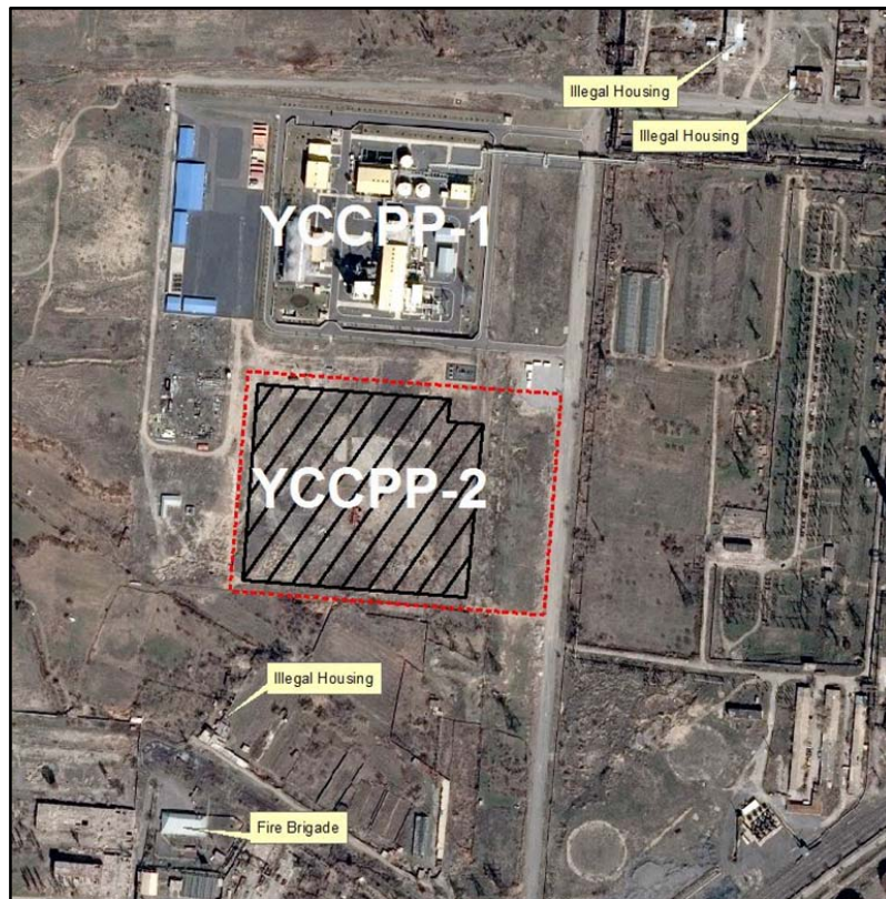
Figure 5-7: Location of illegal houses located northeast and south of new YCCPP-2 and training center of fire brigade
