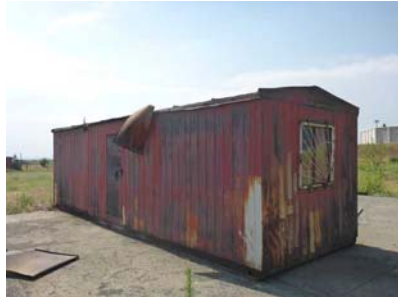
Figure 6-4: Metal cabin on concreted area
