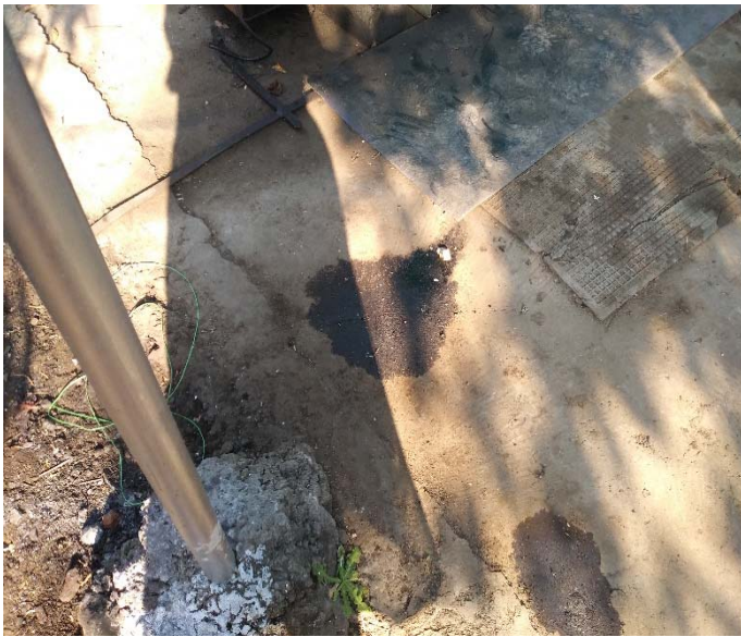
Photo 15: Spillage of oil at D.G. area at Khalghat Toll Plaza
