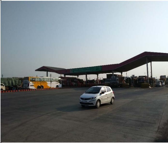
Photo 1: View of Khalghat Toll Plaza
