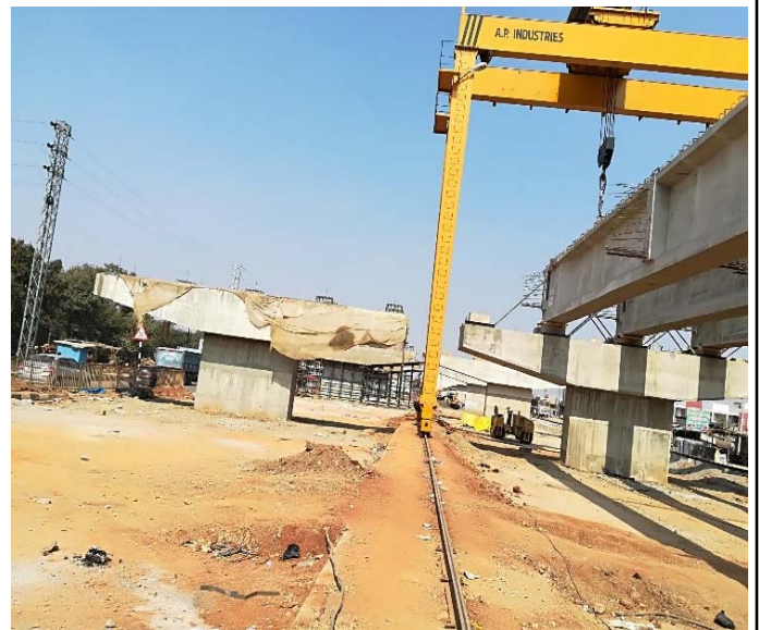
Photo 20: Under Construction Kushtagi Fly Over
