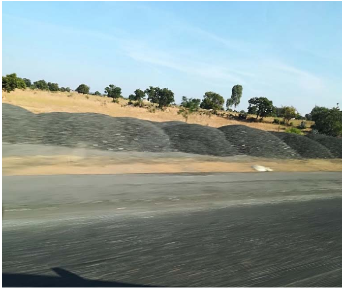
Photo 5: Scarified and Milled Bitumen stored on ROW
