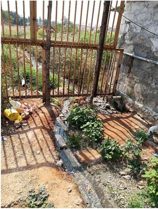
Photo 13: Wastewater discharged on open land at Edoni Camp
