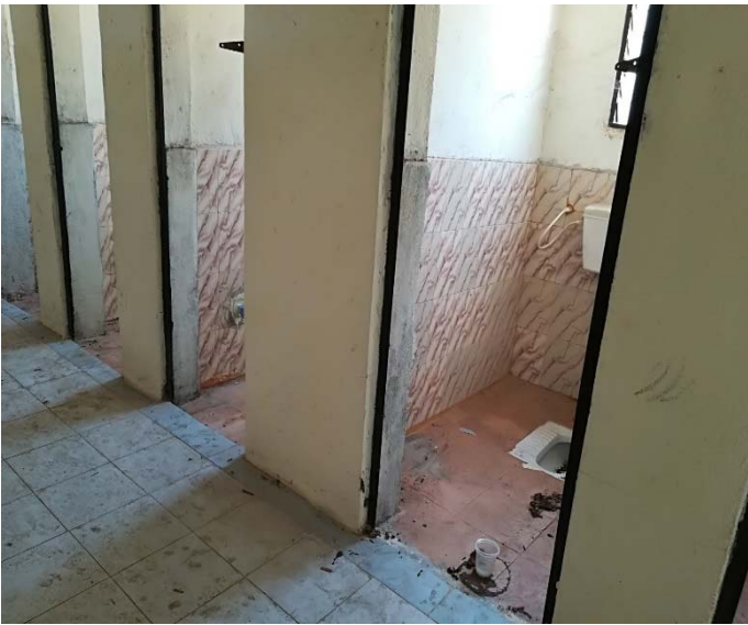
Photo 17: Toilet facility at wayside amenities
