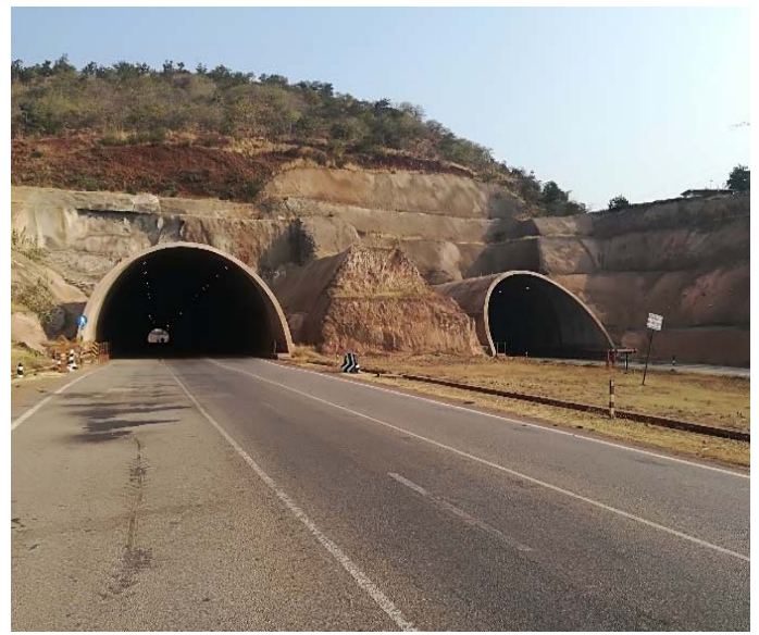
Photo 2: Tunnel at Hospete
