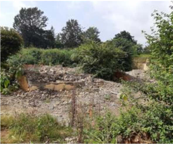
Photo 3: Vegetation around demolished structure.
