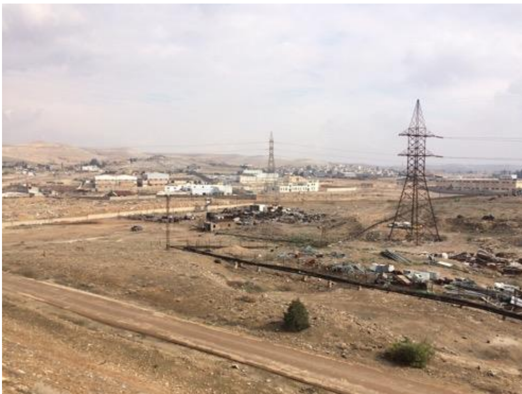
Plate 3-6 Overview of Project Site Sections 1 & 2 (within the internal fence line)
