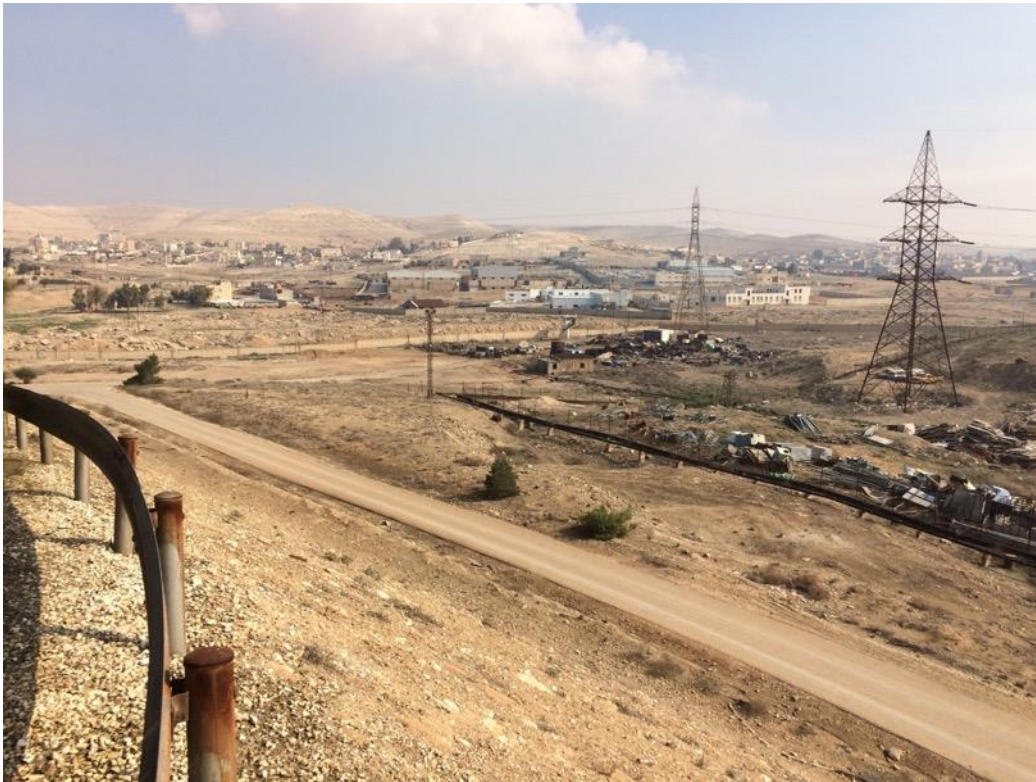
Plate 3-10 Overview of Project Site Section 2 (northern extent – in foreground) – 2016
