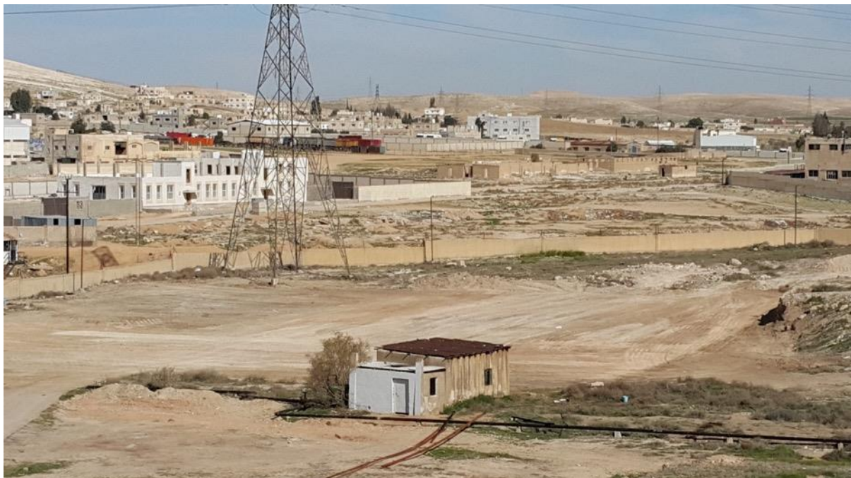
Plate 3-8 View in March 2016 of Site Section 1 – Following Removal of Scrap
