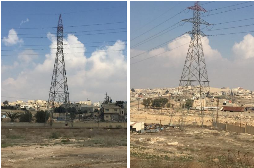
Plate 3-2 Two of the three pylons located in the project footprint
