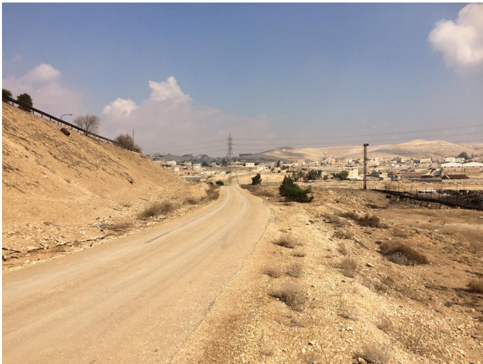
Plate 12-2 Road within Existing HTPS
