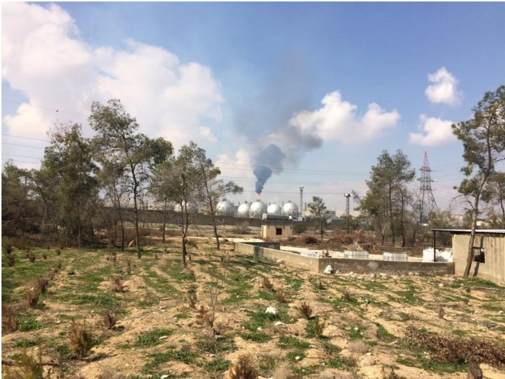
Plate 3-15 Project Site Section 4 with contained chemical storage area (January 2016)
