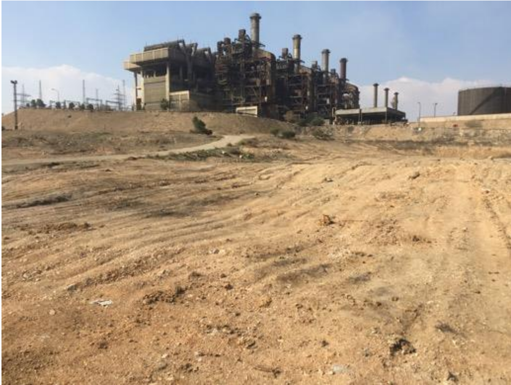
Plate 14-3 View over GT/HRSG/ST Area to the West
