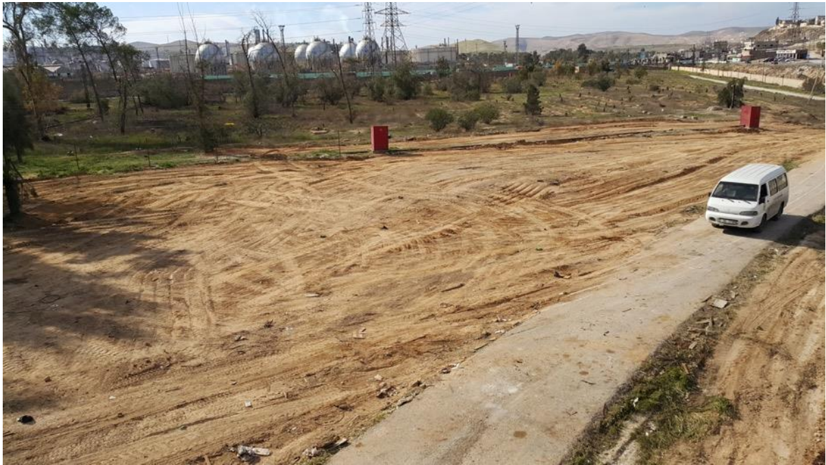
Plate 3-16 Project Site Section 3 – Section of area (March 2016)
