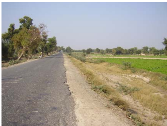
Right of way for pipeline
