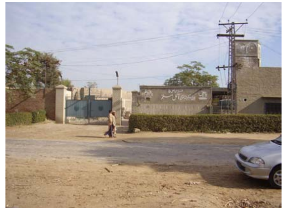
Oil Mill in the vicinity of proposed site
