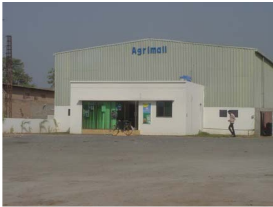
Engro's Farmer facilitation centre under one roof on Sahiwal-Pakpattan Road
