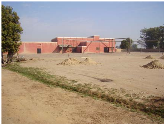
View of distant view of factory at site
