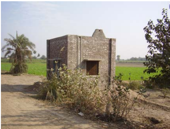
Government tube well installed for water supply
