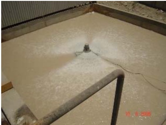
Photograph 4-9: Equalization Basin
