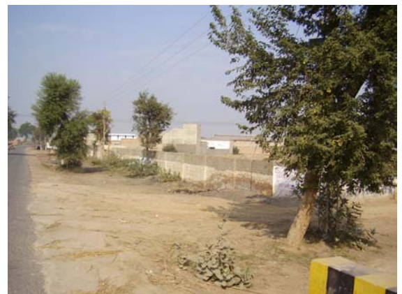
Another view of ROW for pipeline
