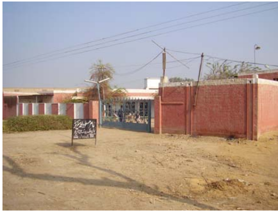
View of existing factory at site
