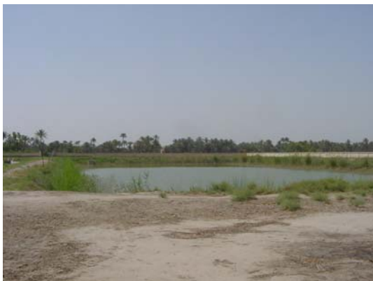
Settling basin for Rohri water supply
