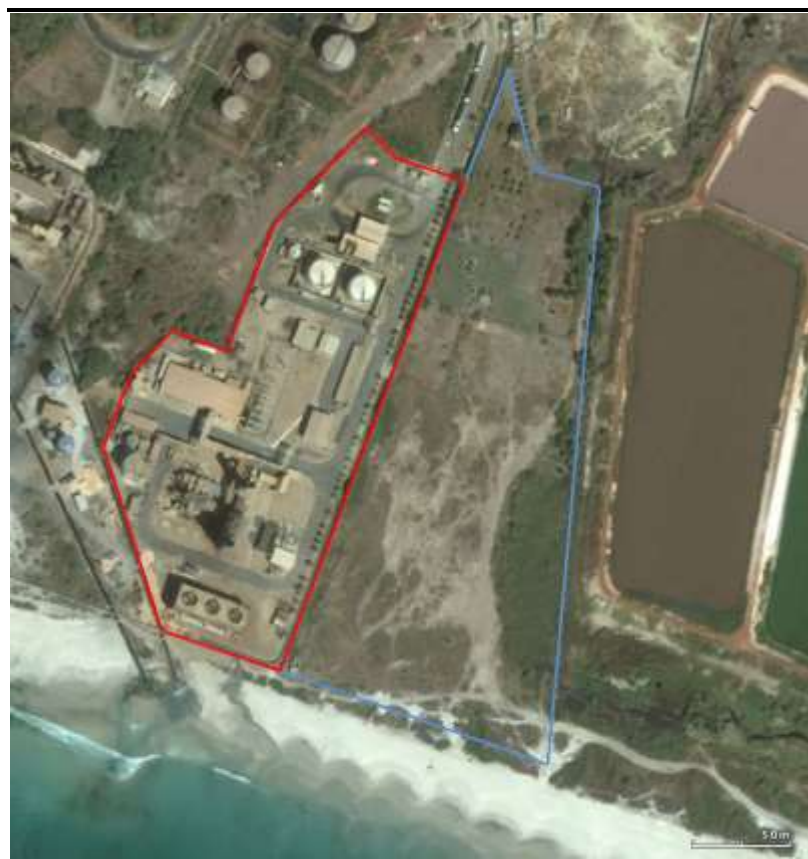
Figure 3.2 Installation site for the 53MW power plant and the 33MW Extension
