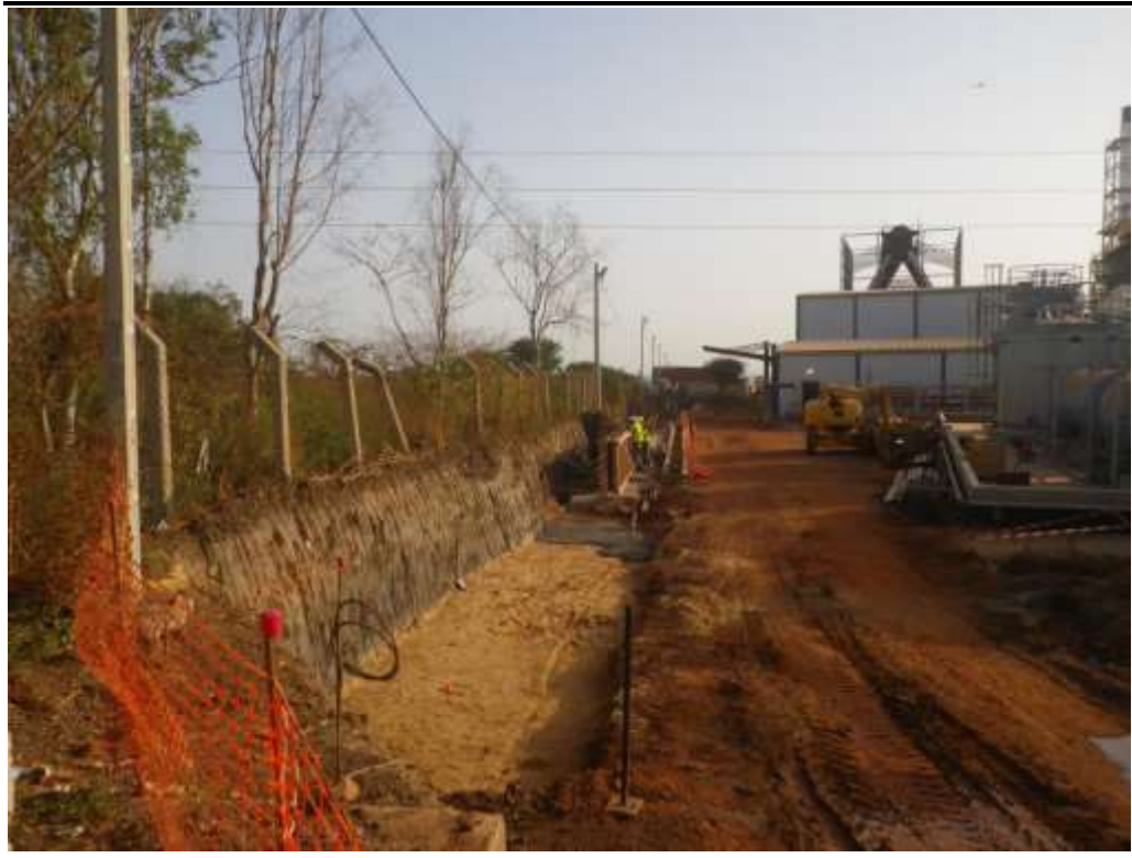
Figure 3.7 Boundary with ONAS Wastewater Treatment Plant: Wall of Pack Dirt
