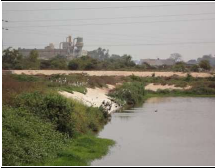
Figure 5.2 Berms around the waste water storage lagoons at the Rufisque WWTP
