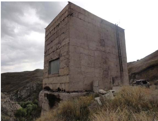
Photo 9: Outlet control building
