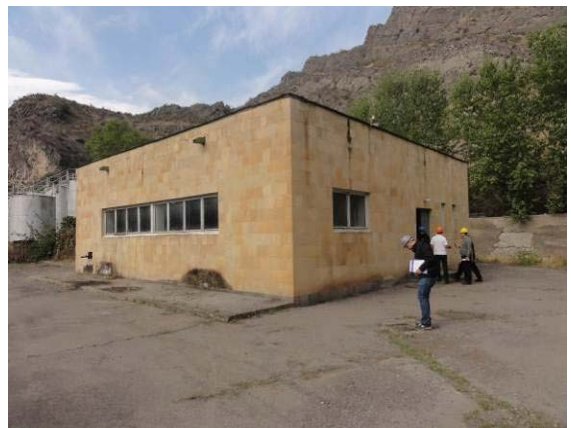
Photo 73: Oil refinery station
