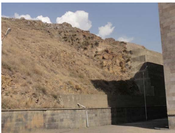
Photo 44: Retaining wall against falling rocks to be extended to both sides and in height
