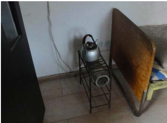
Photo 34: Unsafe heating device
