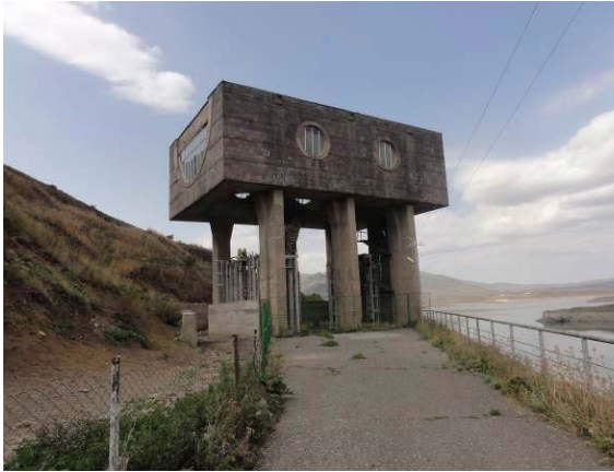
Photo 7: Intake control building
