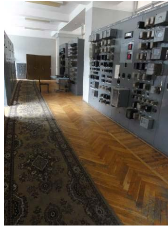
Photo 71: Wooden floor and carpets in control room
