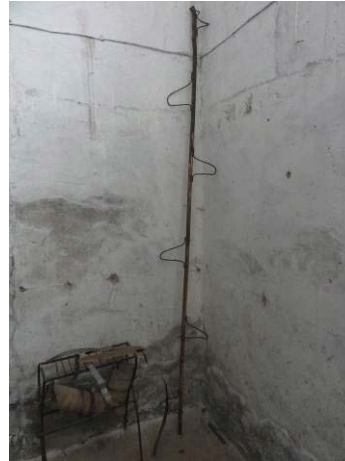
Photo 6: Self-made construction used as ladder
