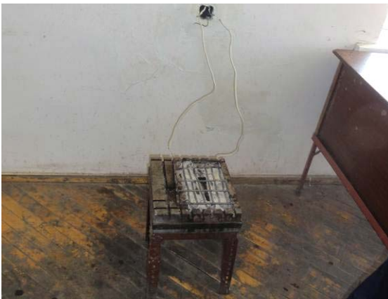
Photo 26: Unsafe heating device
