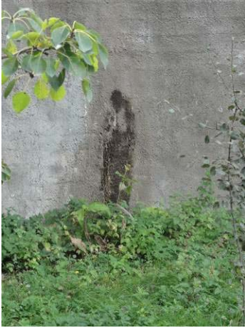
Photo 36: Water leakages at the reservoir walls
