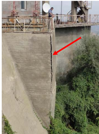
Photo 37: Parts of the concrete walls are breaking off
