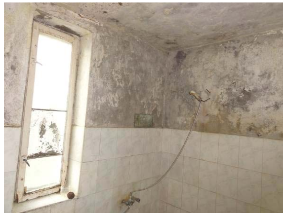
Photo 4: Shower at workers' building
