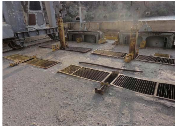
Photo 35: Grids below intake control building
