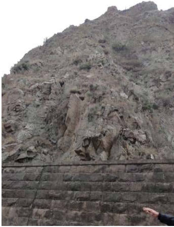
Photo 57: Rocks besides the building
