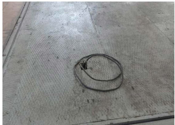
Photo 56: Tripping hazard in machine hall
