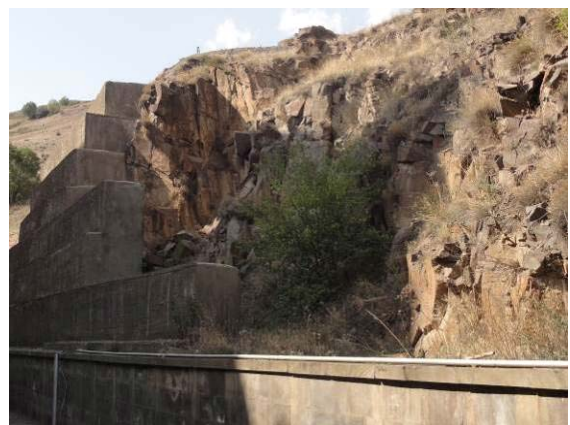
Photo 44: Retaining wall against falling rocks to be extended to both sides and in height
