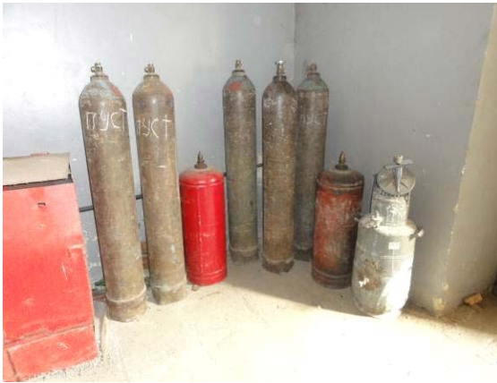
Photo 70: Gas cylinders (some of them filled) not safely stored
