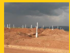
Pile driving work
