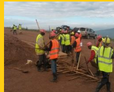
Start of construction
