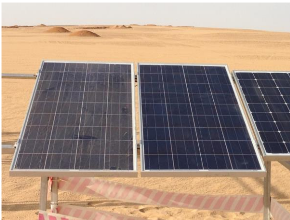
Figure 71: Trial panels at Benban
