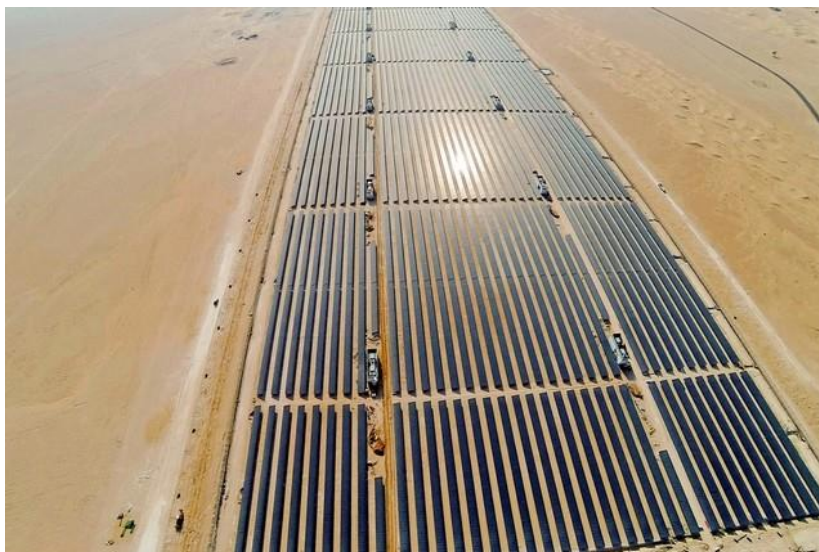
Figure 12. Typical PV Power Arrays Composed of PV Panels
