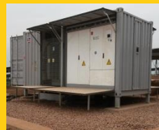
Installation of Inverters
