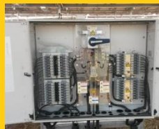
Electrical works / Cabeling
