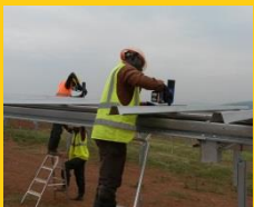
Mechanical installation trackers
