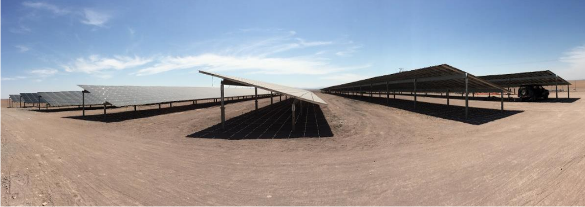
Figure 65. Atacama Pilot PV plant
