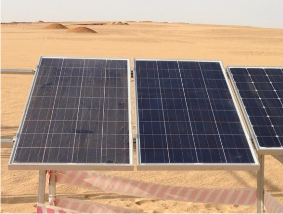
Figure 69: Trial panels at Benban
