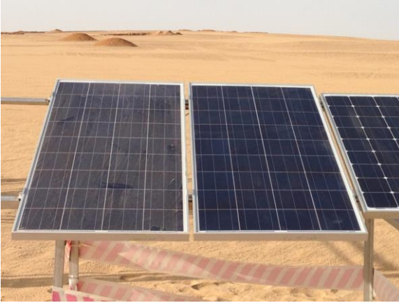
Figure 62: Trial panels at Benban
