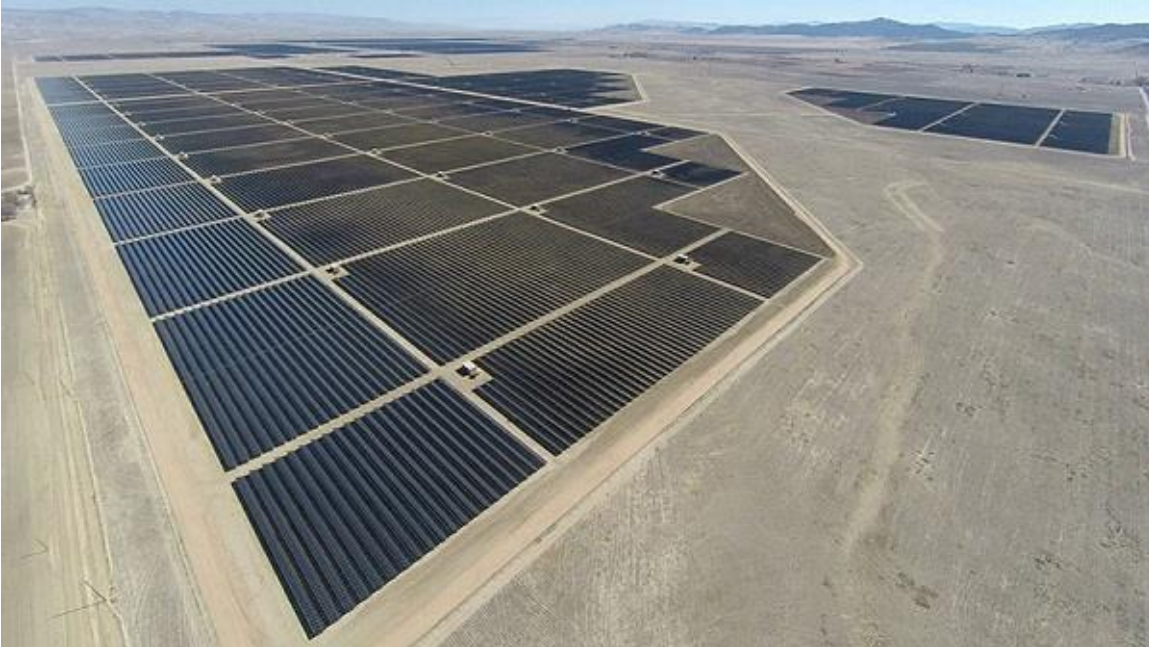
Figure 10. Typical PV Power Arrays Composed of PV Panels
