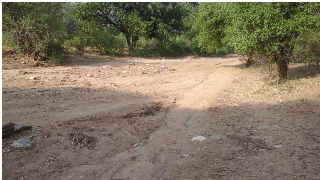
Figure 7.1. Gully formation along exiting track inside the project area
