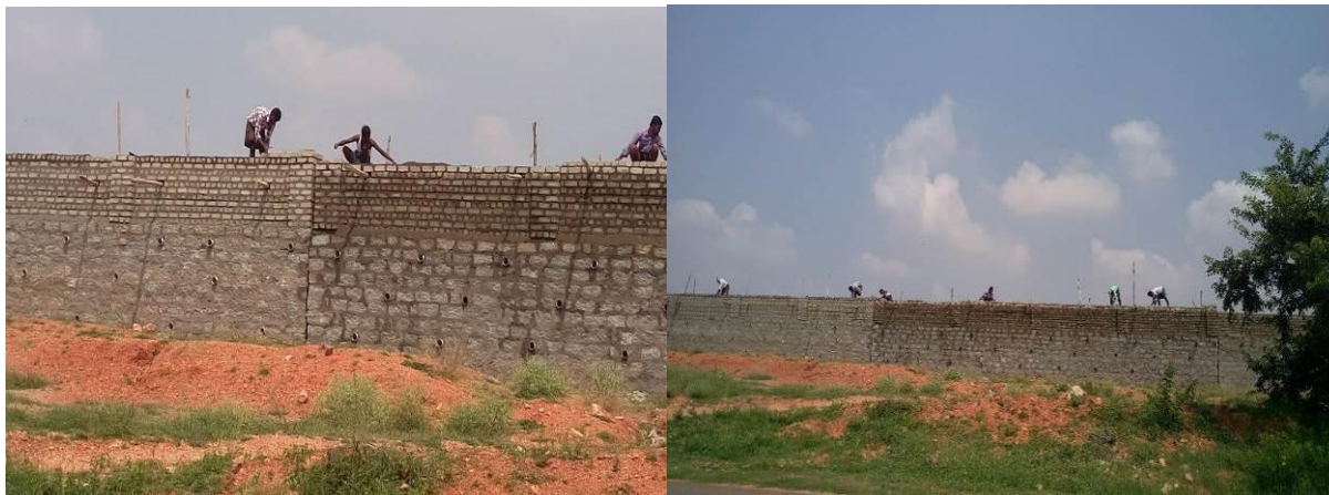
Photo-Grid Substation under construction
