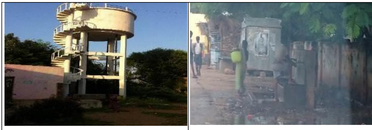
Photo- Drinking Water Facility in study area villages
