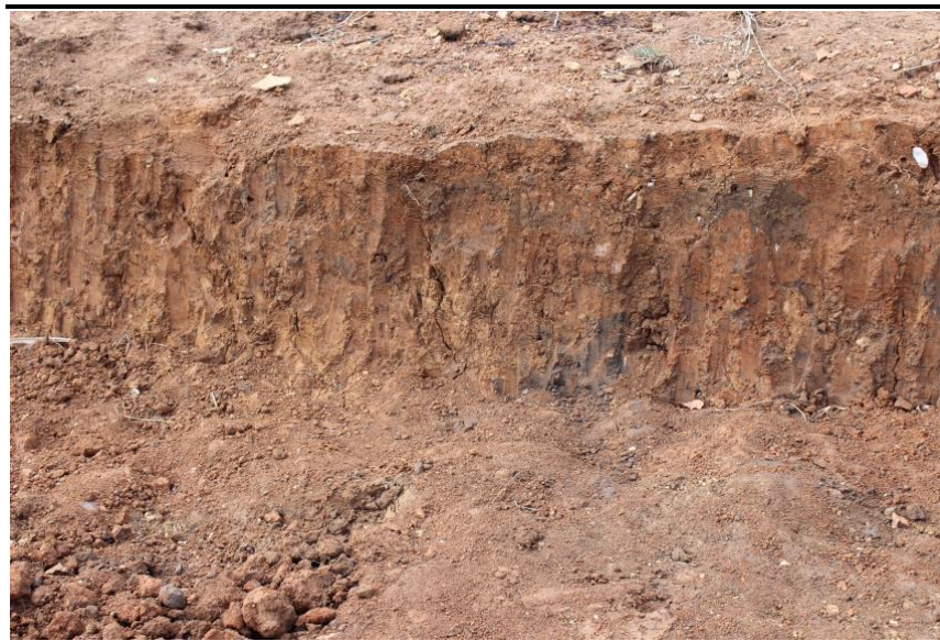
Figure 4.38 Vertical cuts existing in several points of the project area
