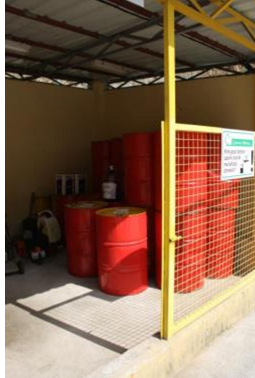
Photo 2: Otluca HEPP - Oil storage compound – good practice (no spill kit present).
