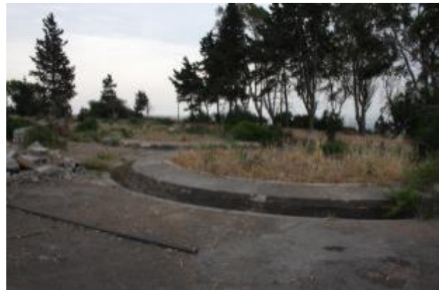
Photo 8: Mercin CCGT Site: Plinths for redundant former oil tanks.
