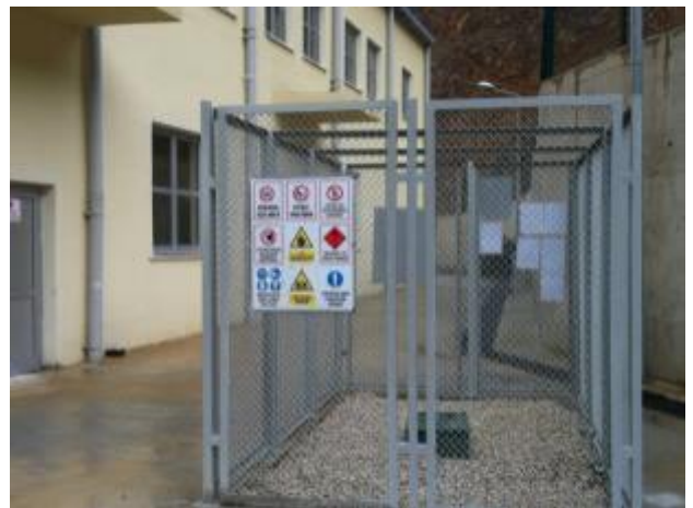
Photo 14: Doruk HEPP - LPG storage.
