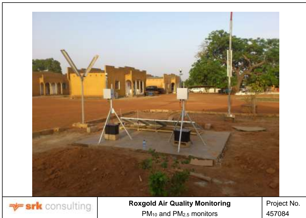
Figure 5-3: PM 10 and PM 2.5 monitors installed at the Roxgold Mine Camp.
