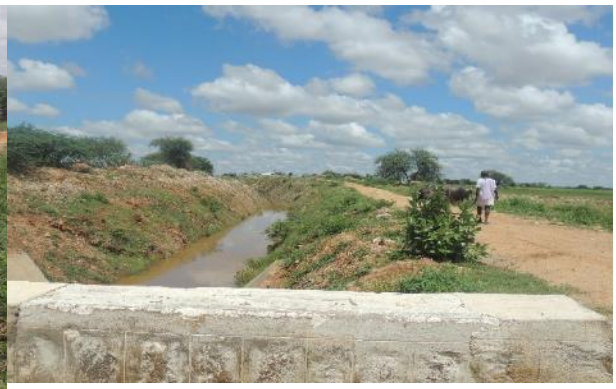
Unlined canal running north of project site approx. 6 km away
