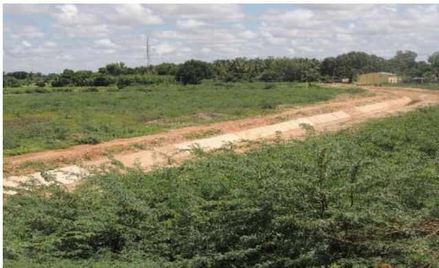
Canal connecting Vedavati river to Challakere
