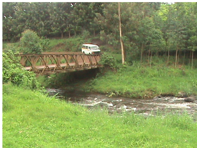
Plate 5 The bridge near the proposed intake along river Kiringa
