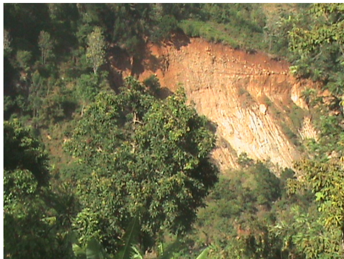
Plate 8 The proposed powerhouse site close to the landslide prone area
