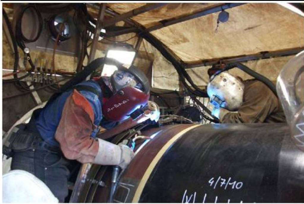
Figure 4.27 Example of Pipe Welding
