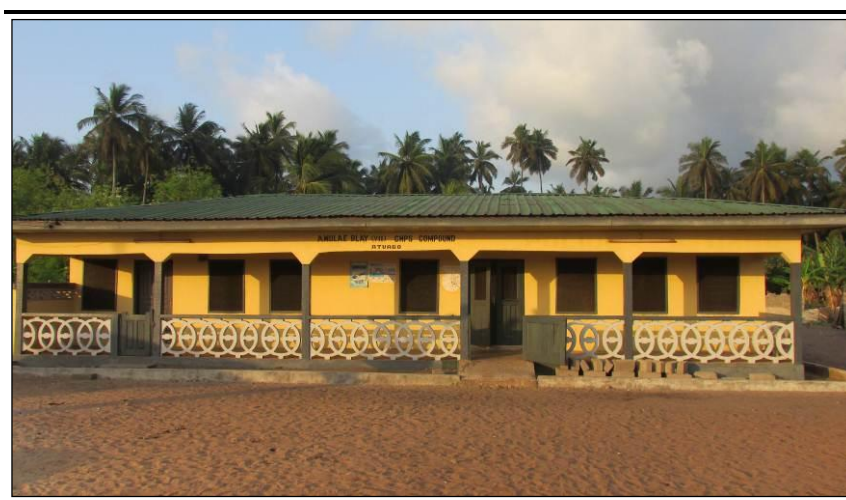
Figure 9.3 Atuabo CHPS Compound, 2014
