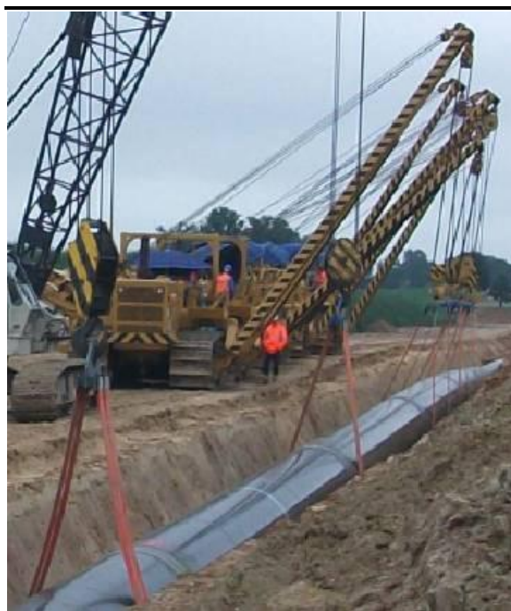
Figure 4.29 Example of Pipe Lowering
