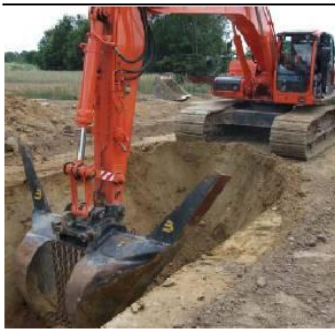
Figure 4.28 Example of Pipe Trench Excavation
