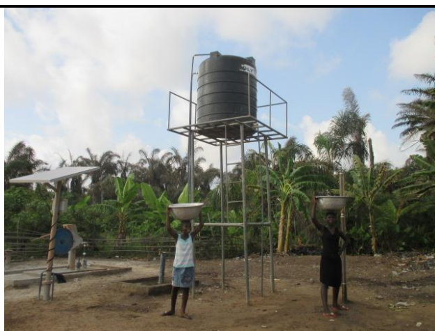
Borehole working with solar system in Sanzule
