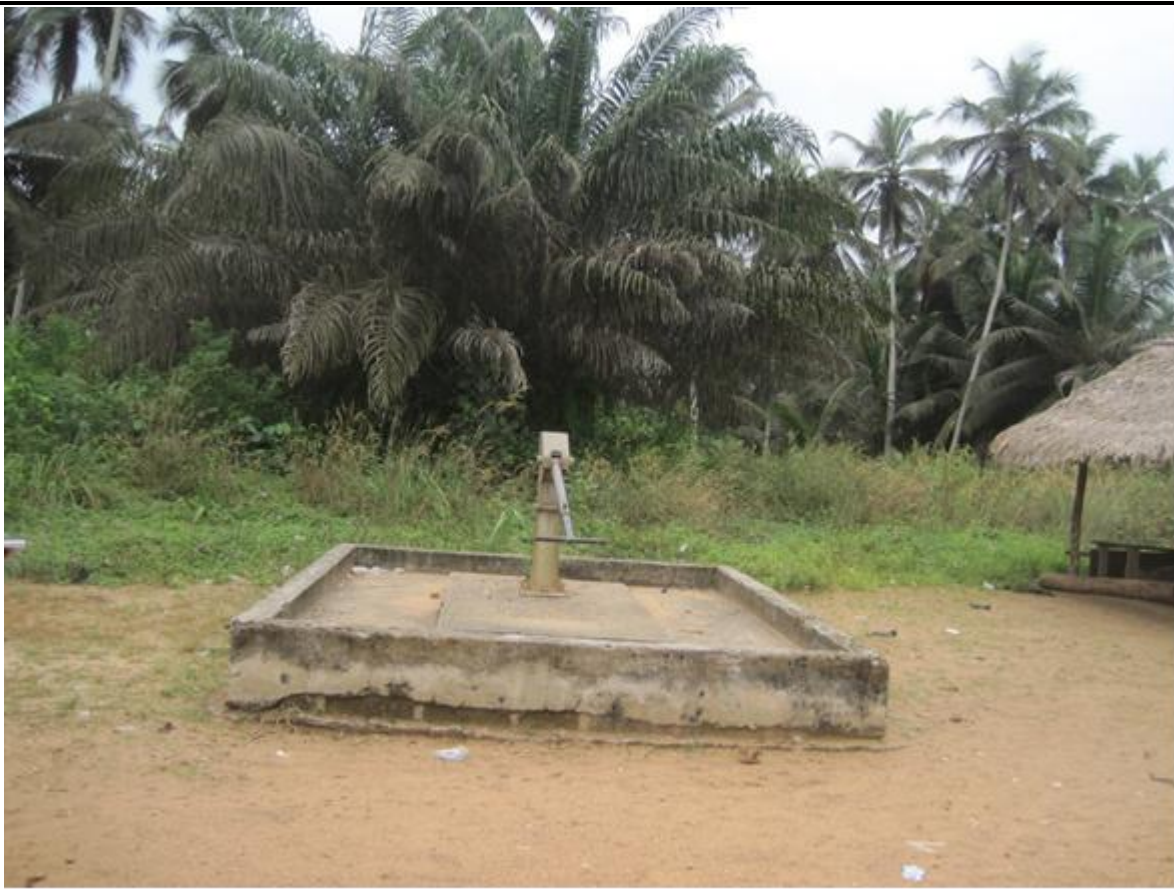
Figure 8.12 Typical Bore Hole and Associated Hand Pump in the DAoI
