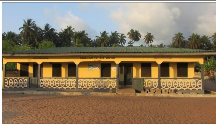
Figure 6-3 Atuabo CHPS Compound, 2014
