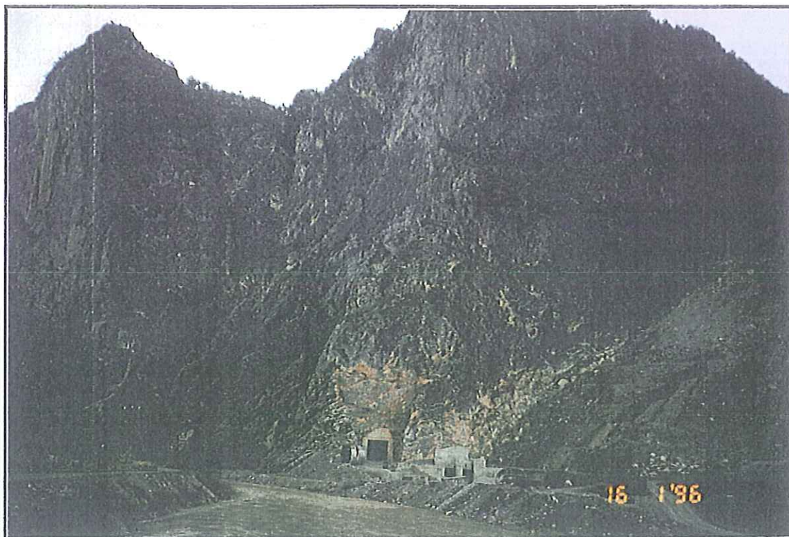
Photograph IV.1. The Diversion Tunnel Entrance
