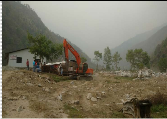
Photo 26: Land Clearance activities being undertaken at Khalte site
