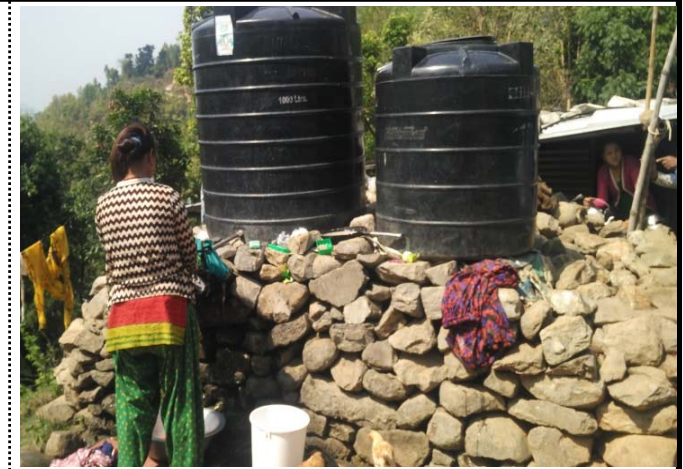
Photo 9: Water Facilities in Bogetitar IDP Camp
