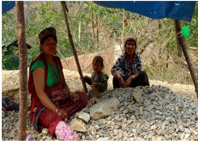
Photo 13: Stone Breaking activities in Dhunche
