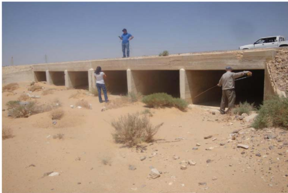
Figure 45: Ma'an and Al Mdawwara Road Culvert near the project Site
