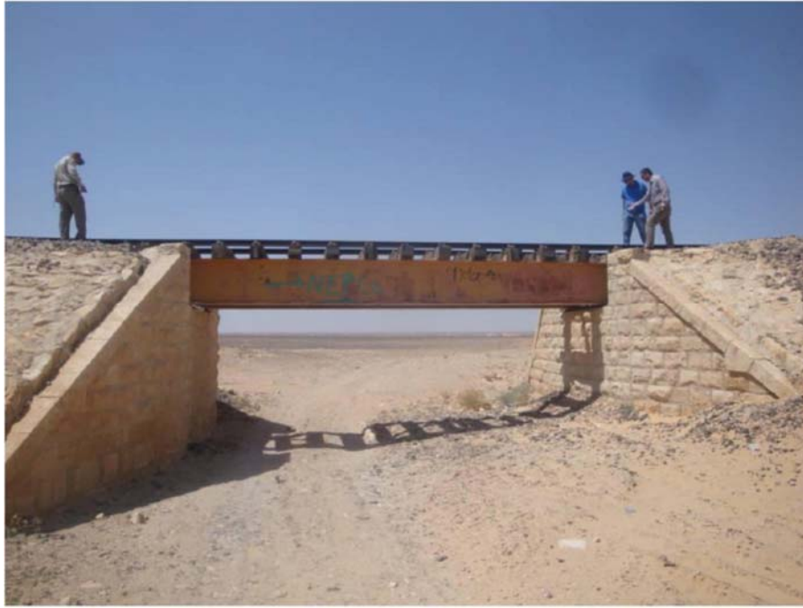
Figure 44: The Al Hejaz Railway Bridge near the project site
