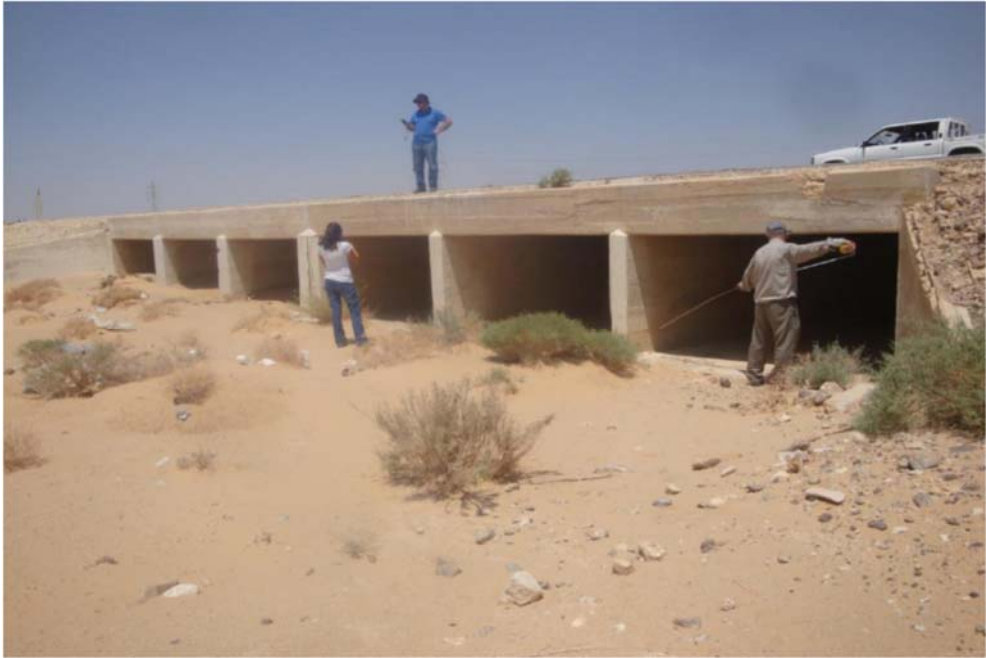
Figure 39: Ma'an and Al Mdawwara Road Culvert near the project Site.
