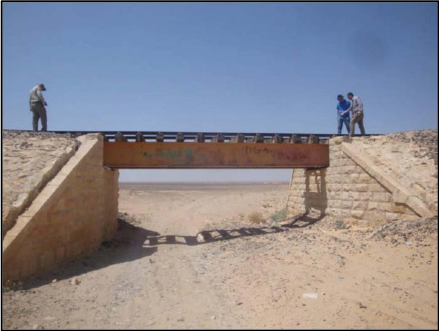
Figure 38: The Al Hejaz Railway Bridge near the project site.
