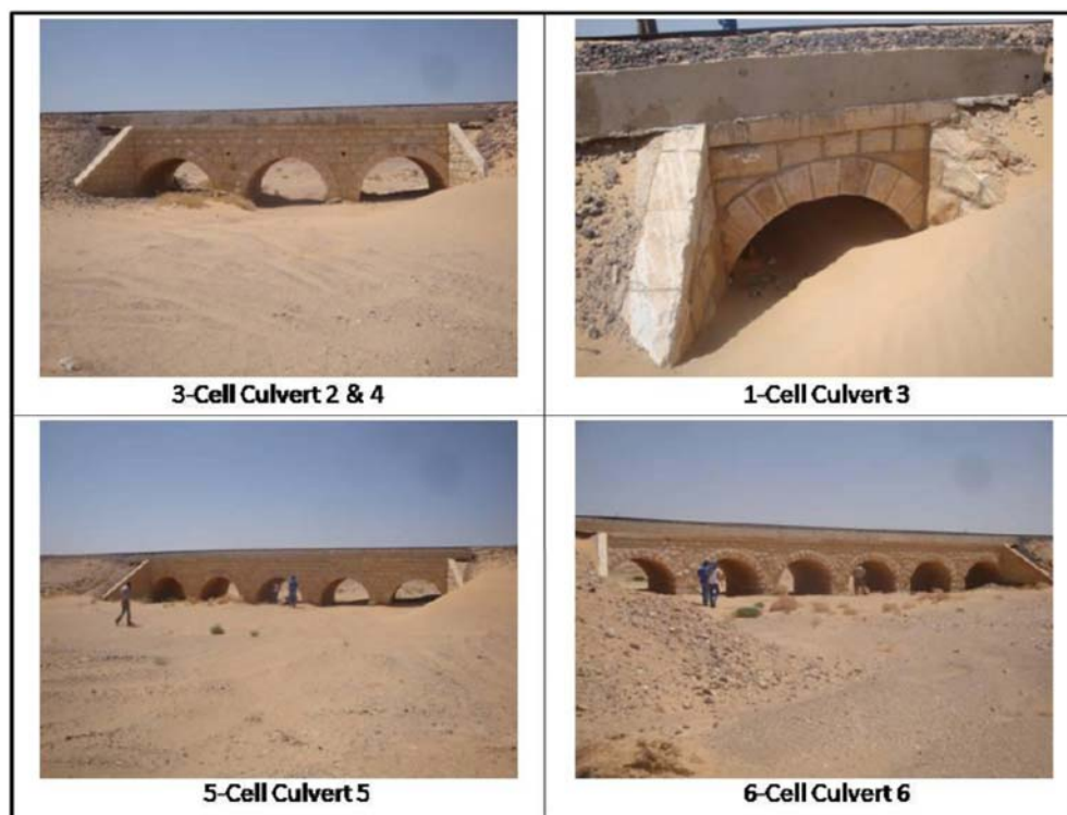
Figure 37: Culverts observed in the project site.
