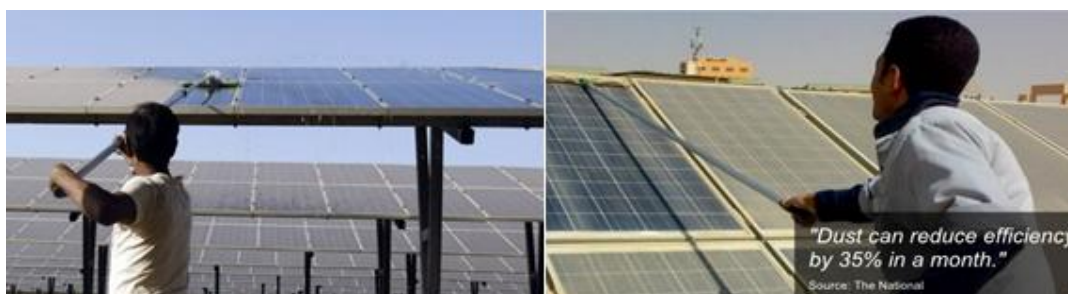
Figure 21: Cleaning of Shamsuna PV modules will be done through a dry brush cleaning programme (Cube, 2014)
