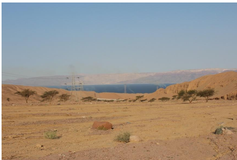
Figure 32: Acacia raddiana trees across the wadi of the transmission line (ECO Consult, 2014)
