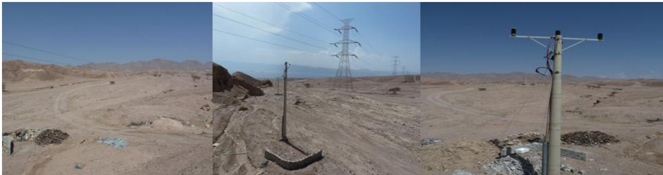
Figure 19: Photos of Existing Wadi 2 Overhead lines (Cube Engineering, 2014)
