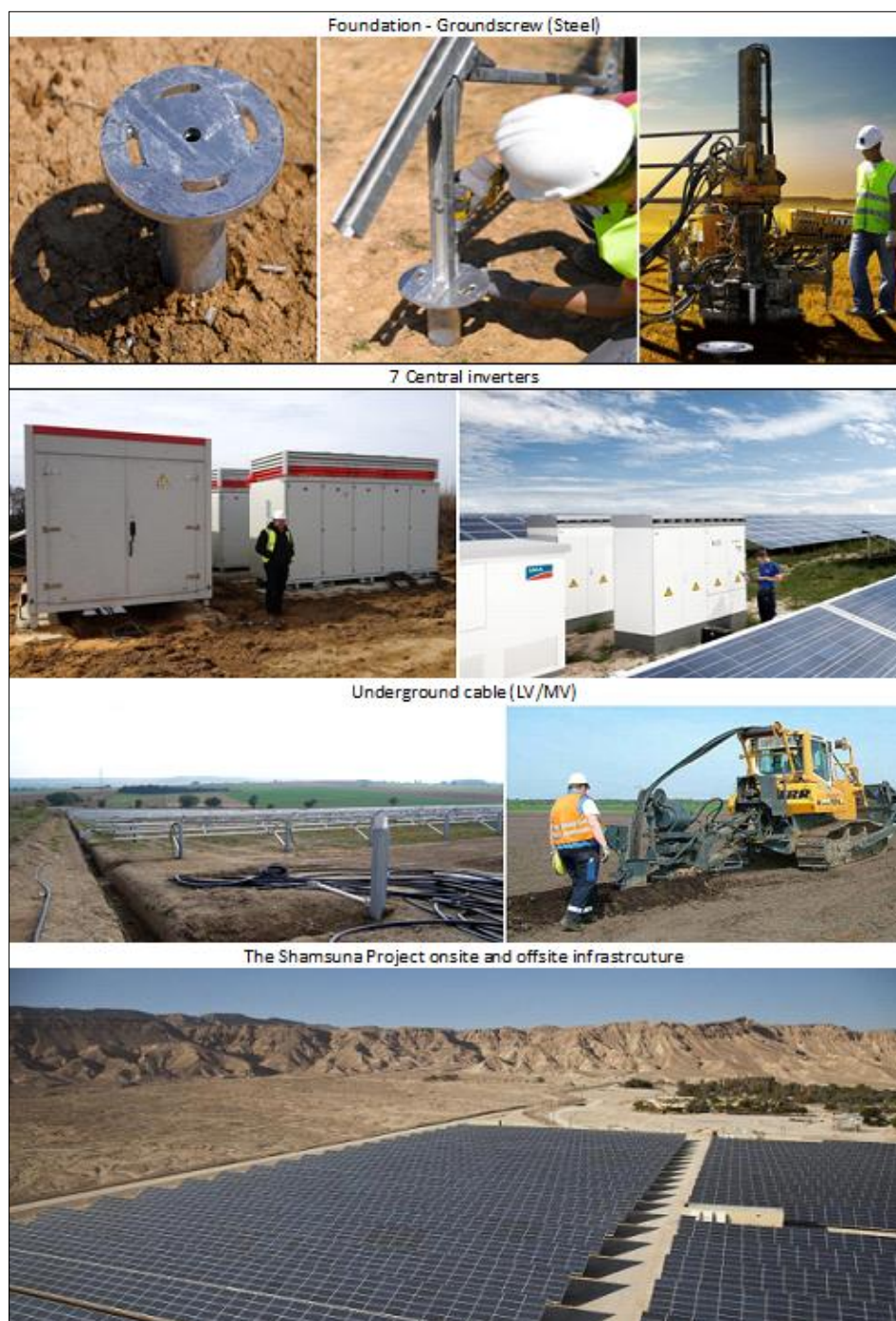
Figure 20: Typical activities during the construction phase for PV farms (Cube Engineering, 2014)
