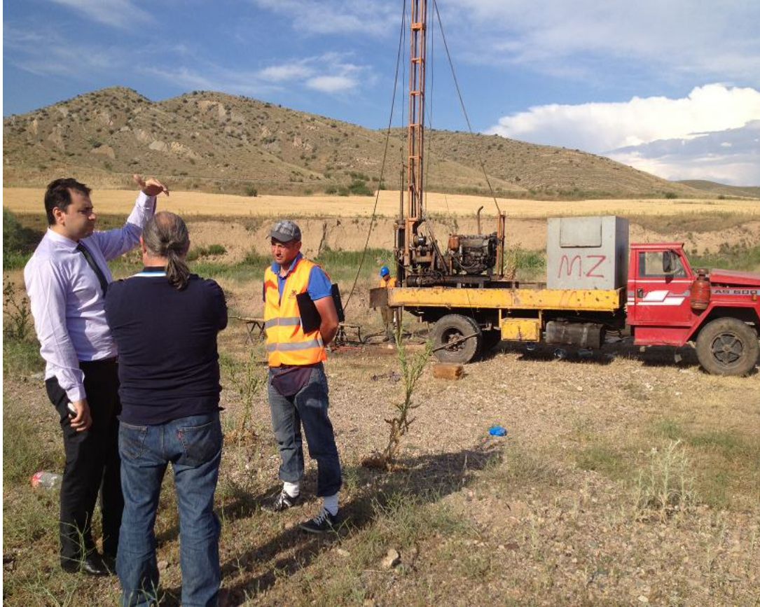
Figure 32. SK-10 Drilling Works
