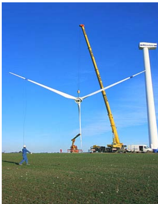
Figure 3.16 Installation of Nacelle and Blades
