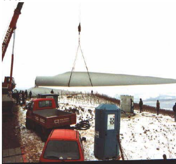
Figure 3.15: Assembly of Rotor Blades
