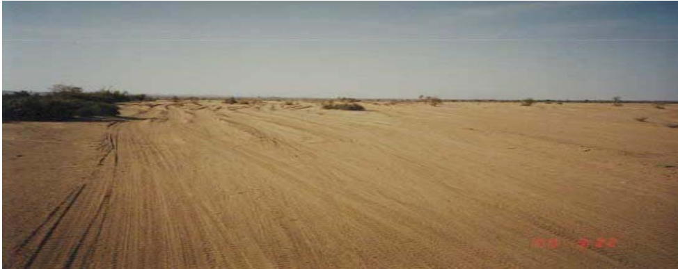
Figure 4.8: The road in Deh Kohistan showing the numerous paths taken by vehicles.
