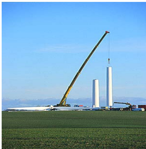
Figure 3.14: Installation of Towers
