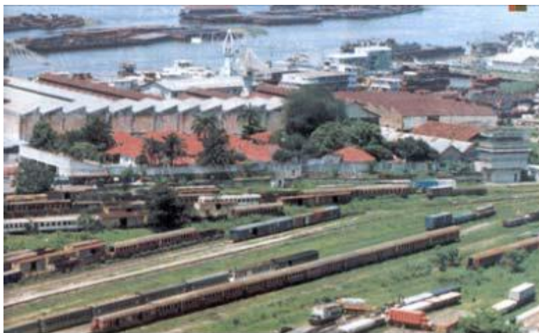
Figure 4-20: Aerial view of railway marshalling yard
