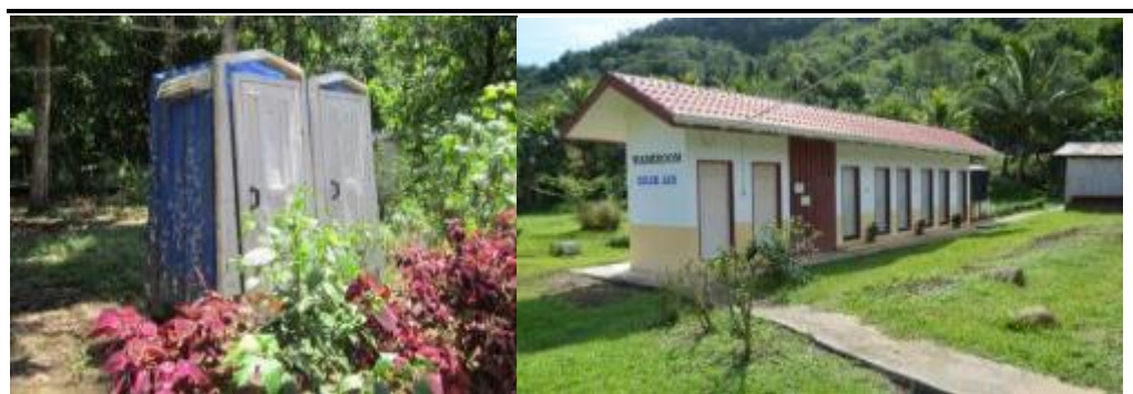
Figure 5.33 View of Sanitation Facilities
