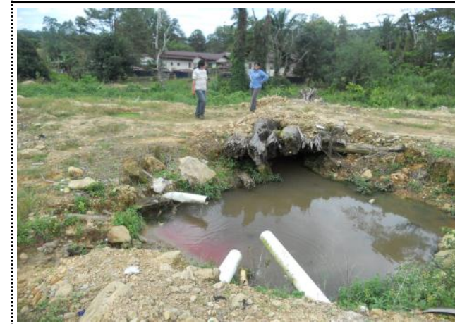
Photo 30: Effluent discharge pond at the Nepali worker camp in Mendulong
