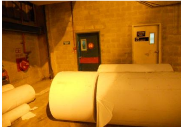
Photo 13: Obstruction of fire exit at PnP shop floor
