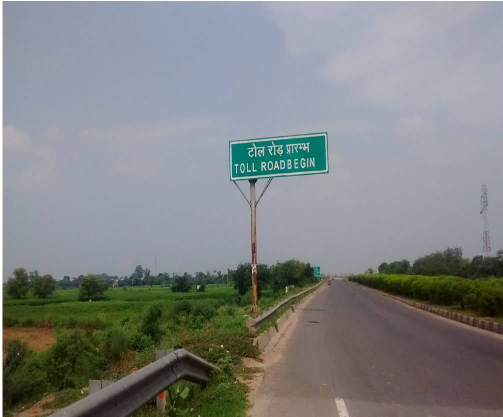
Photo 5: View of Toll Road board at project starting point
