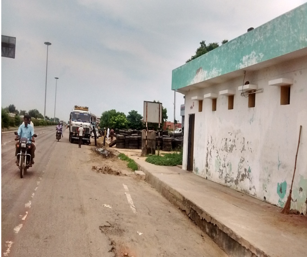
Photo 21: View of the encroachments falling within the ROW
