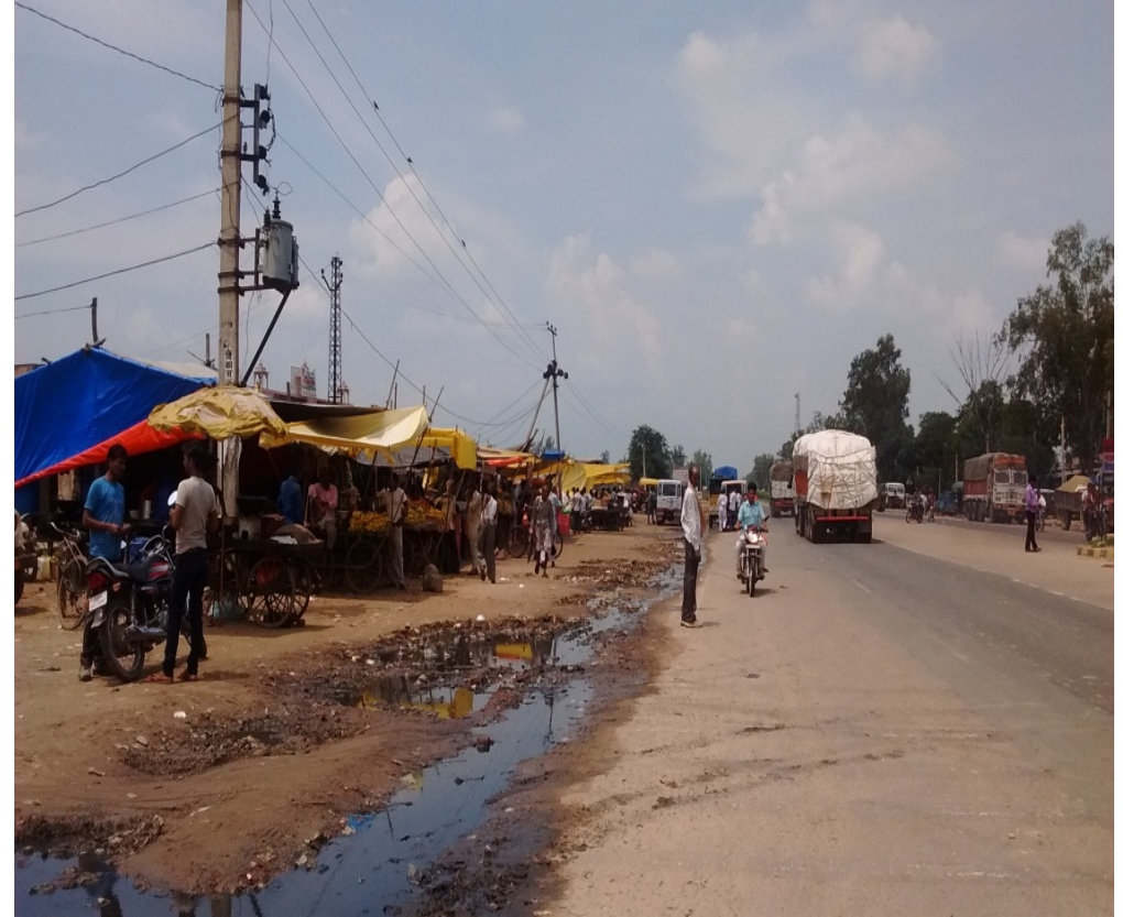
Photo 26: View of the poor maintenance of carriageway.
