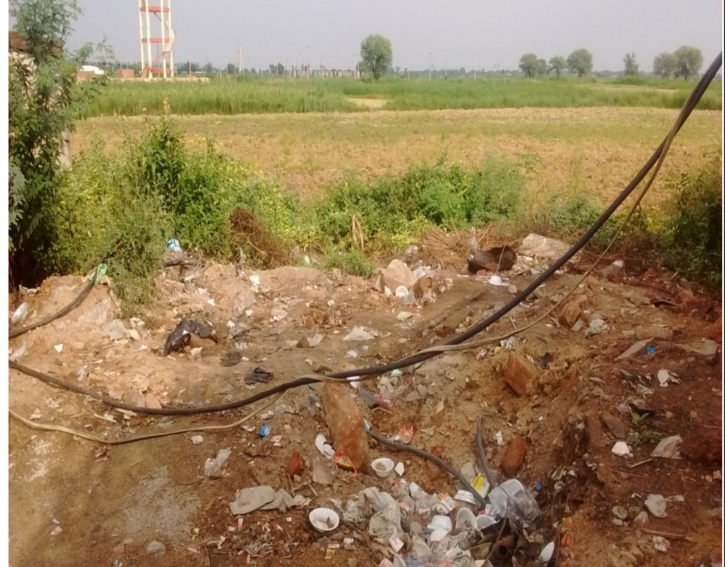
Photo 4: View of the poor ROW maintenance with no solid waste management
