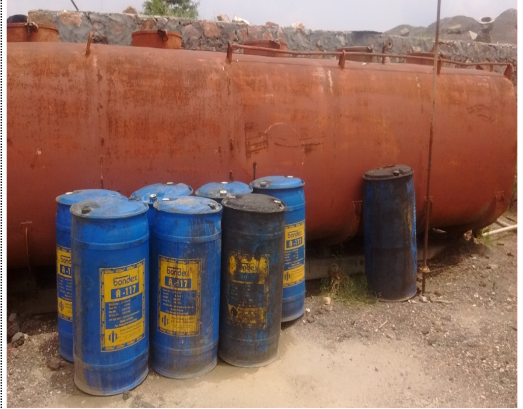
Photo 16: View of the diesel barrels directly exposed to land without any secondary containment
