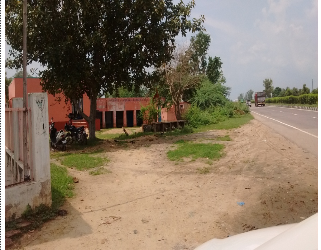
Photo 14: View of the primary school falling within the ROW as an encroachment and no structural barrier and safety measure implemented.
