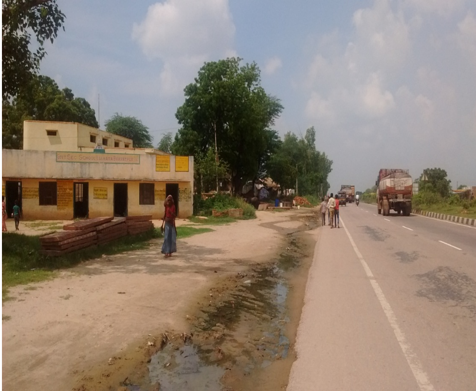
Photo 13: View of primary school without an structural barrier, falling within the ROW, is also an encroachment and no ROW maintenance.
