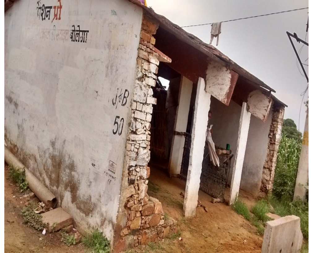
Photo 22: View of the encroachments falling within the ROW
