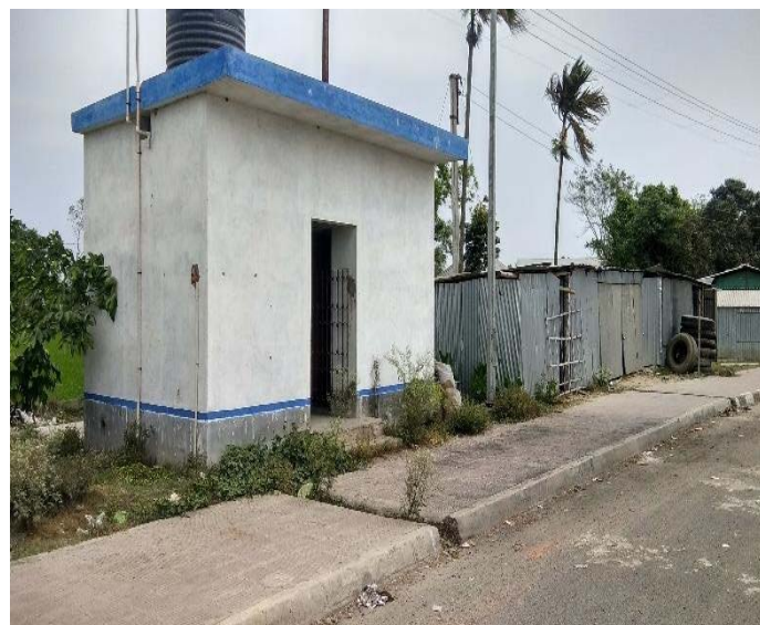
Photo 26: Toilet at truck lay bye
