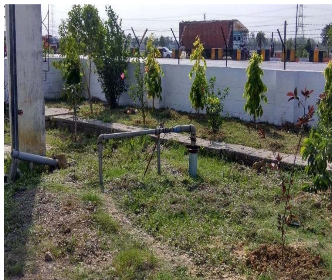
Photo 24: Bore well at toll plaza
