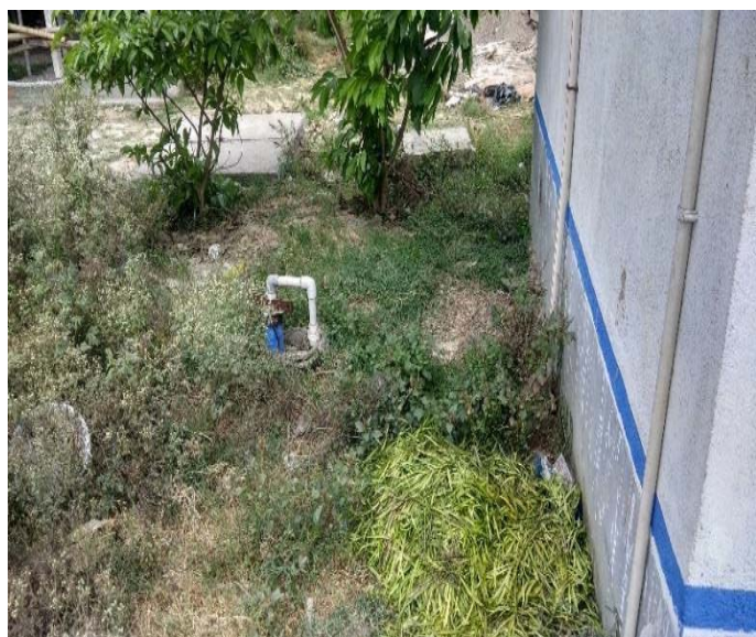
Photo 23: Bore well at labour camp
