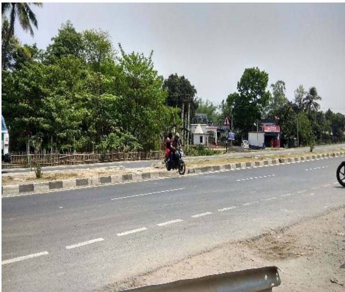
Photo 31: Unauthorized median opening
