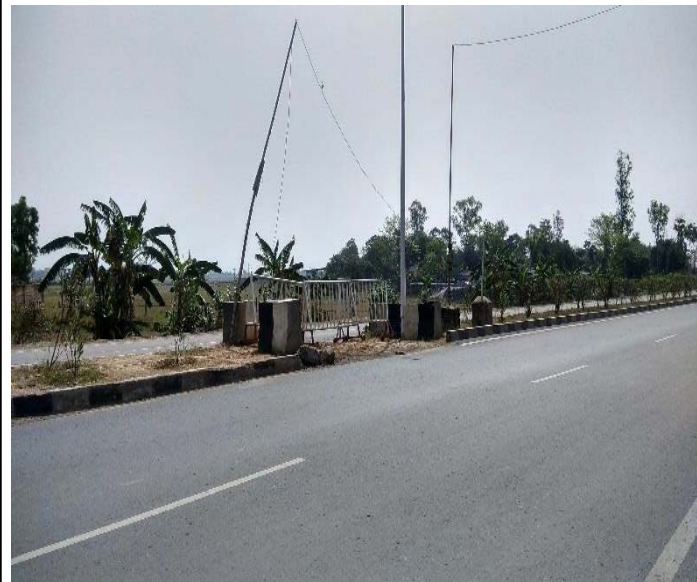
Photo 32: Unauthorized median opening temporarily blocked by road maintenance team
