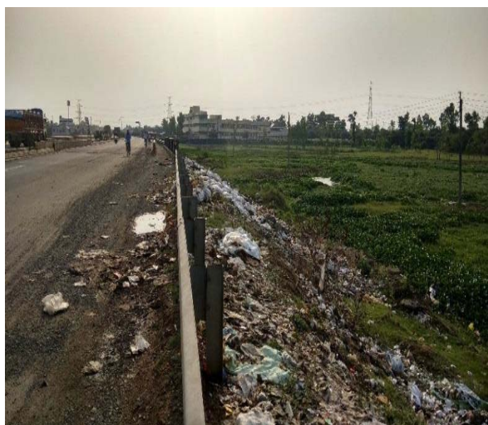
Photo 21: Solid waste within the ROW of project road
