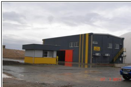
Photo 5. Medical waste sterilization unit
