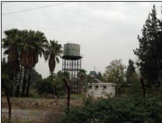
Photo 5. Elevated water tank inside DSI area
