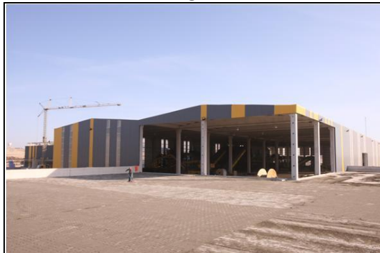
Photo 1. Waste sorting unit
