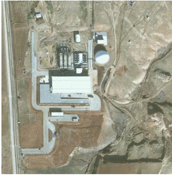
Figure 8-1: AISWDF facility (Source: Adana Provincial Environment Report, 2011)
