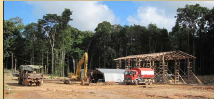
Maintenance Facility (under construction) and Equipment
