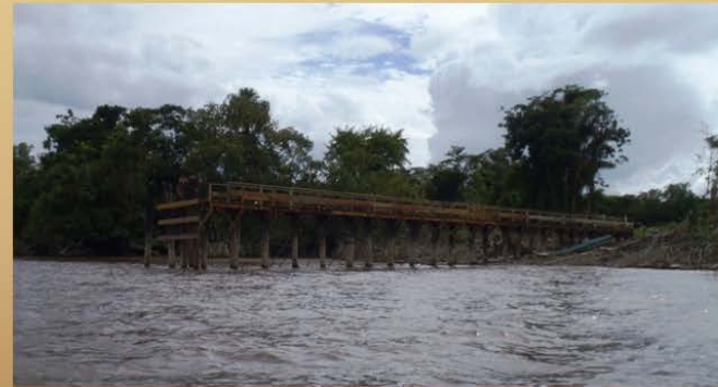
Fuel Unloading Pipe Trestle
