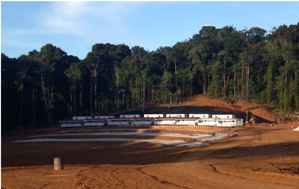
Figure 2.2-4: New Modular Man-Camp Under Construction, Aurora Site (2012)
