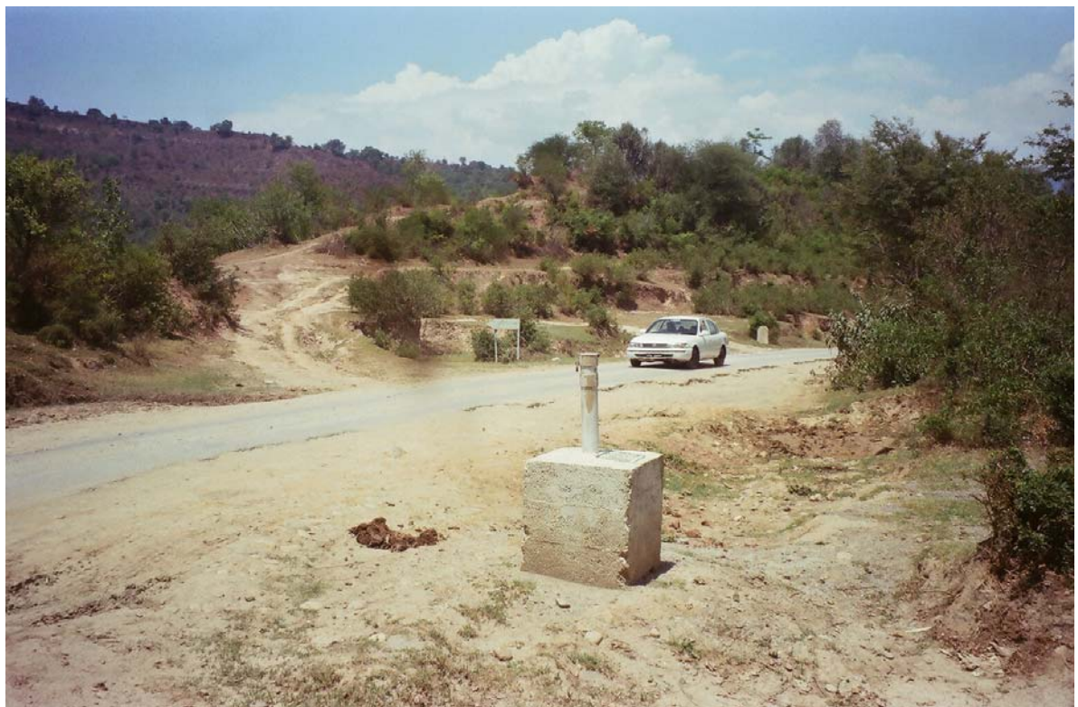
Kahuta-Karot-Kotli Road (With graveyard and Test Borehole area)
