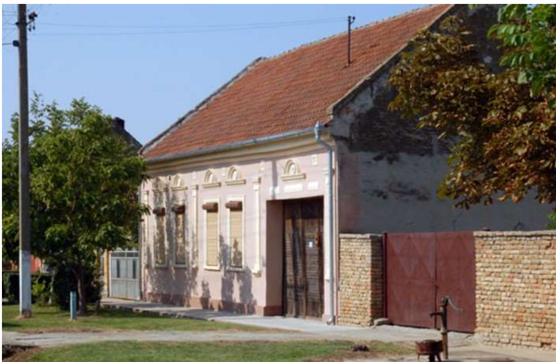
Figure C.12: Photograph: Typical house in local communities surrounding the Project site.
