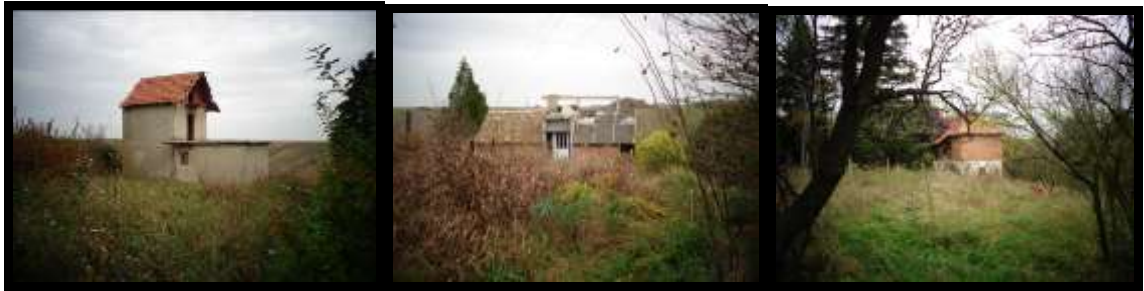
Figure D.3: Derelict Buildings (A, B and E) to the North of Mramorak
