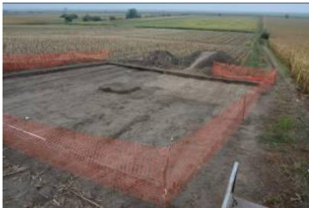
Figure11: Base after the removal of the surface layer
