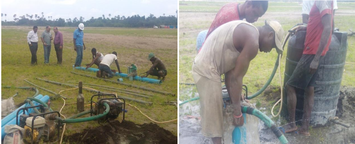
Plate 4-5: Borehole drilling at the fertilizer site
