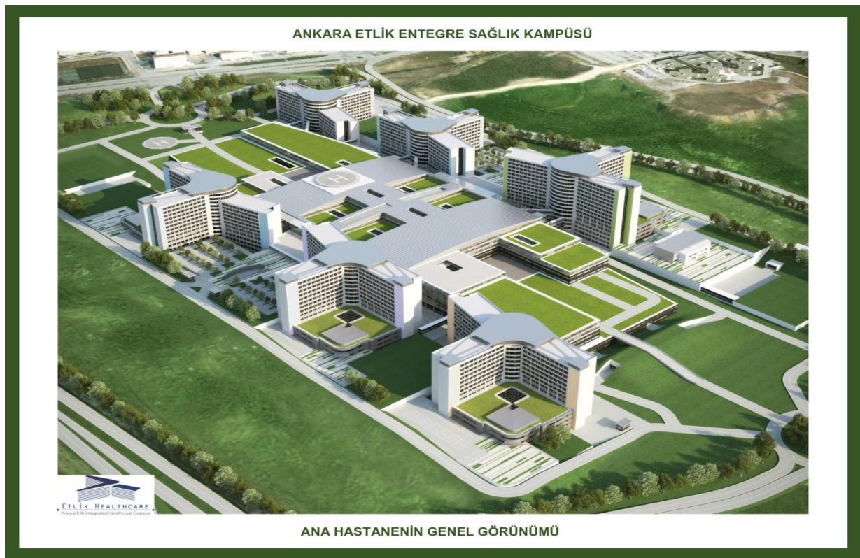
Figure 2-7. General View of the Core and the Towers
