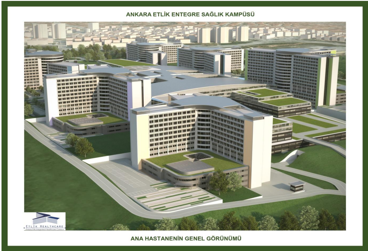
Figure 2-8. View of the Core and the Towers (T3 in front)
