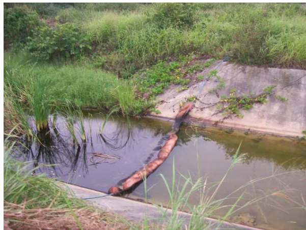
Plate 12: Typical oil absorbent pad in an open drain at TTPS
