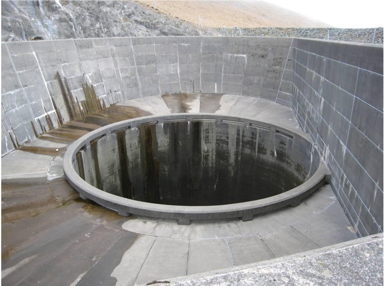
Figure 2.12: Example of surge shaft
