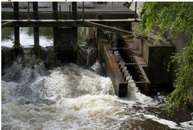
Figure 2.11: Examples of different fish pass structures
