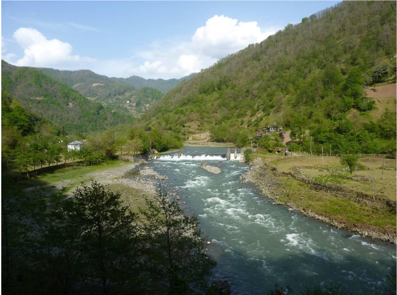
Figure 2.9: Existing Machakhlistsqali HPP Concrete Weir
