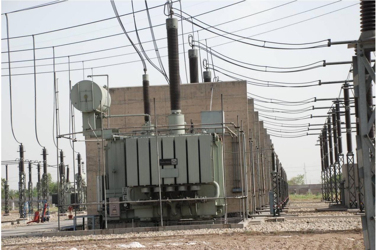
Figure 2.16: Example of Transformer and Switchyard location
