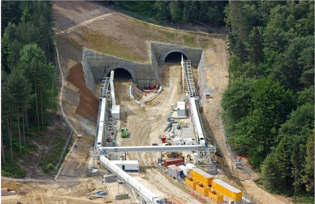
Figure 2.13: Example of Tunnel and Portal Construction
