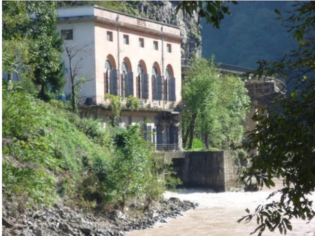
Figure 2.14: Existing Asti HPP Surface Powerhouse
