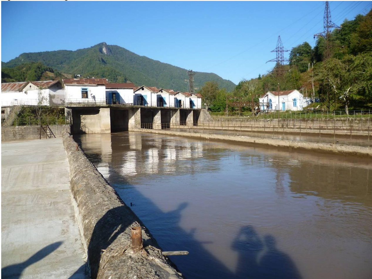
Figure 2.10: Existing Asti HPP Sediment Basin
