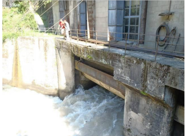
Figure 2.15: Existing Asti HPP Tailrace
