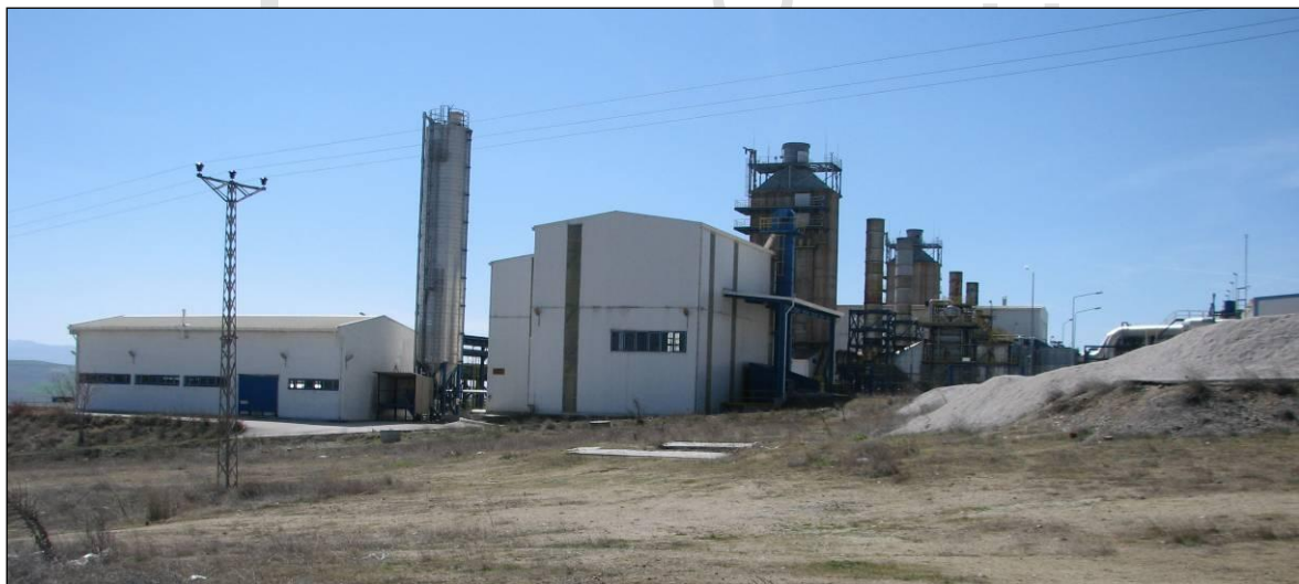
Figure 3-7 BARMEK GAMA Power Plant
