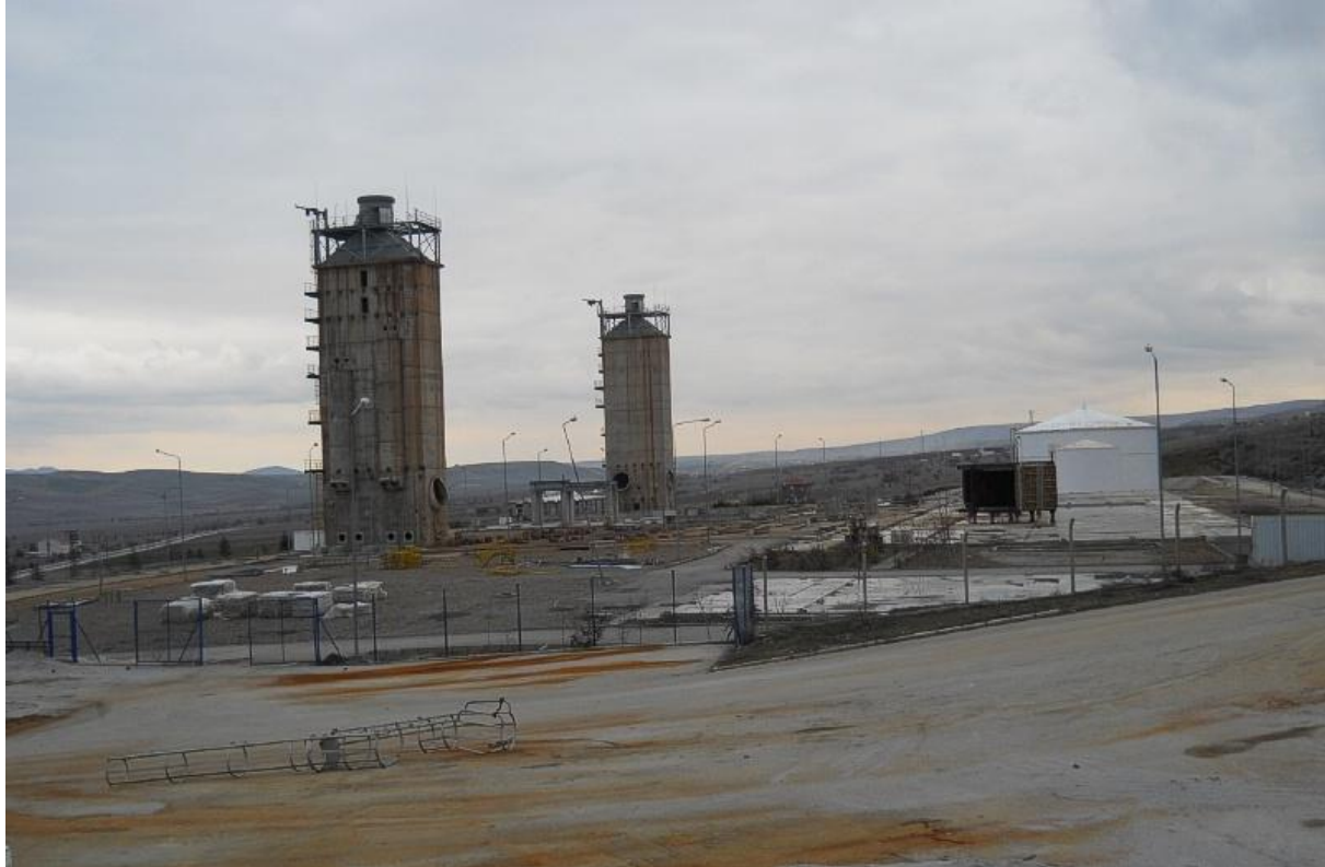
Figure 3-8 BARMEK GAMA Power Plant Area After Disassemble
