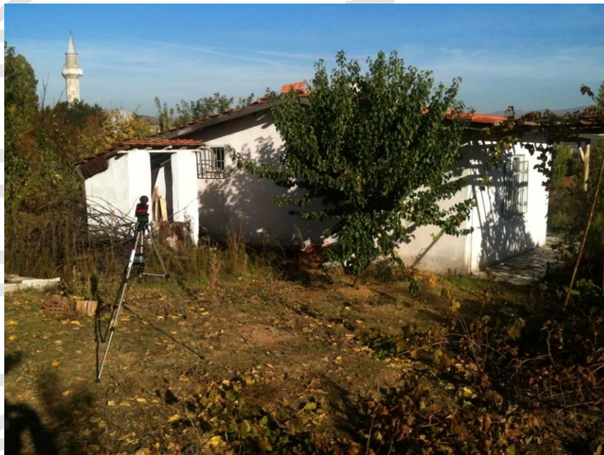
Figure 4-14 View of NSR-1
