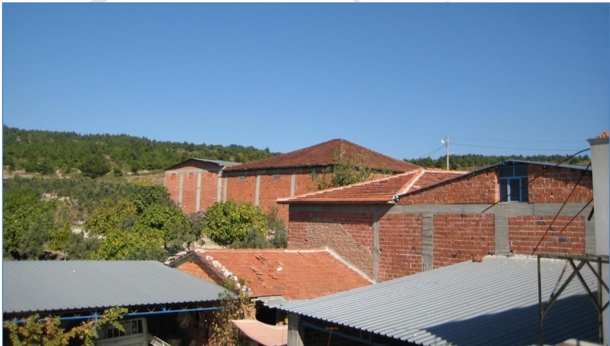
Figure 4-4 View of NSR
